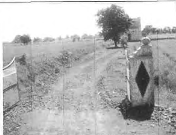
Scarified bitumen waste utilized in approach road at 27.006 RHS.
