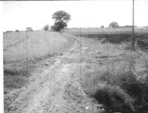
Scarified bitumen waste utilized in maintenance of village approach road at 29.350 LHS.
