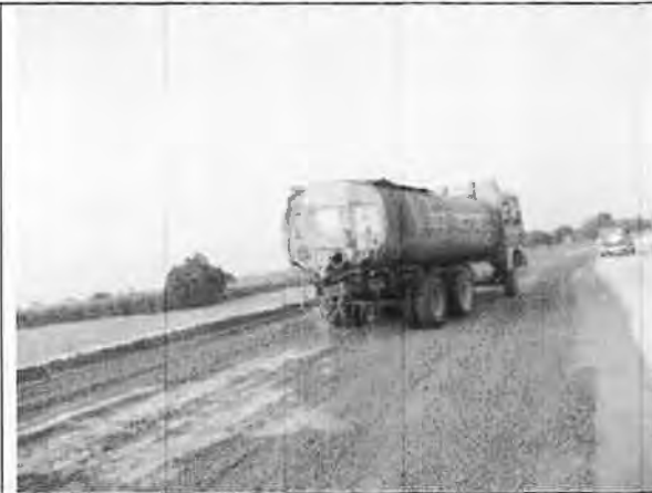
A view of water sprinkling at site for minimization of dust pollution
