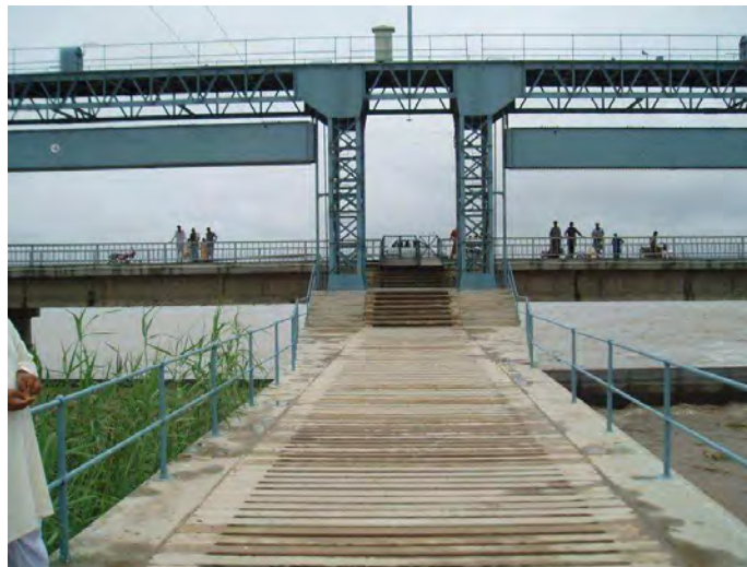
Fish Ladder Located along the divide wall
