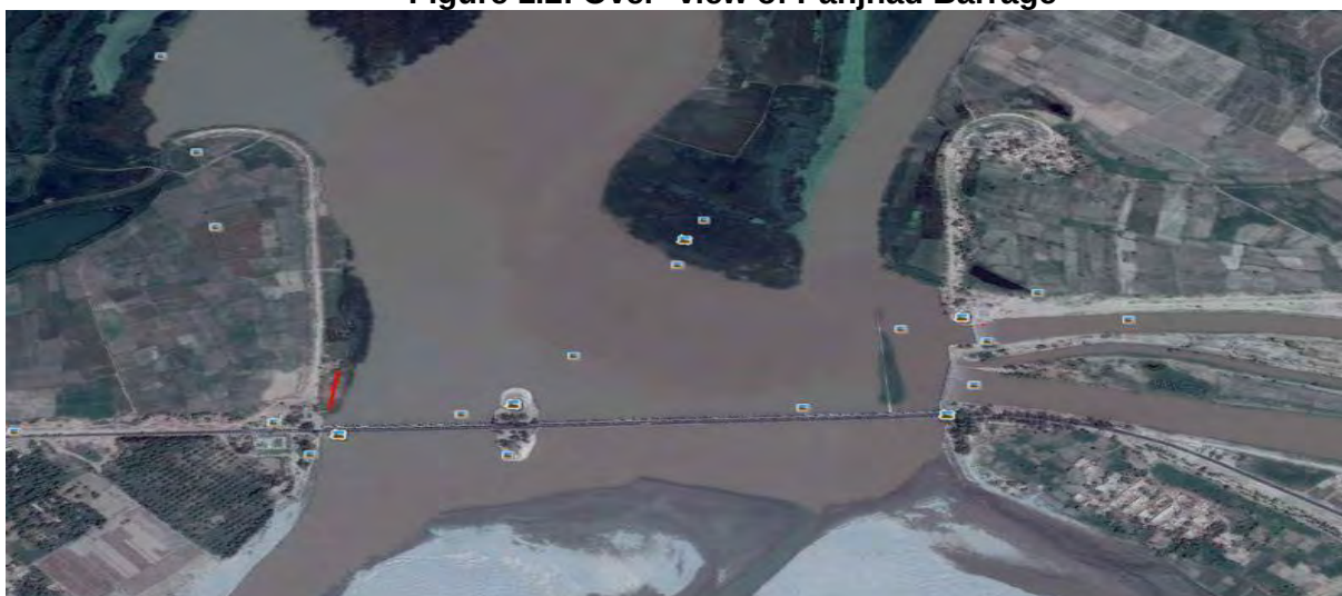
Figure 1.2: Over- view of Panjnad Barrage
