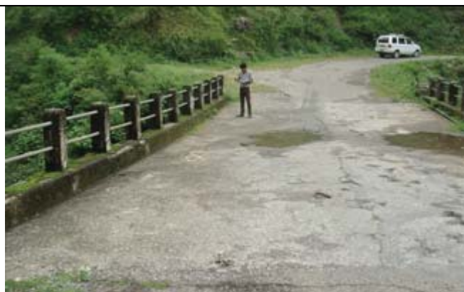
1 Raipur-Kaddukhal Motor Road,Bandal khad, C.H.-7.7
