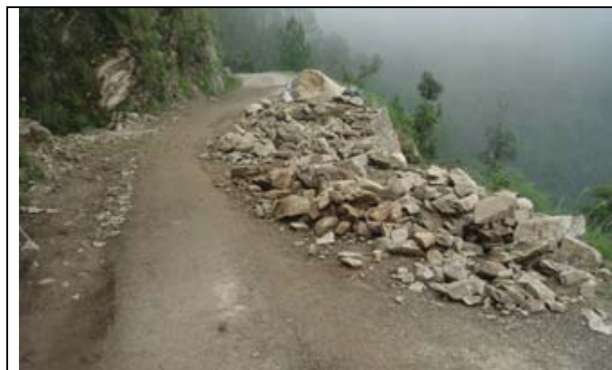
1 Raipur-Kaddukhal Motor Road,Bandal khad, C.h.-39.3
