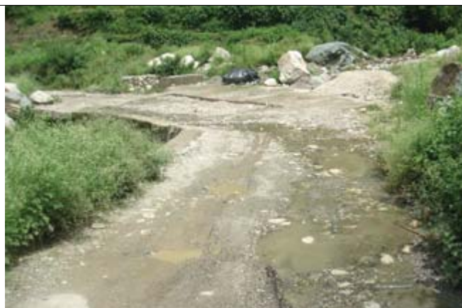
3 Ghansali Tehri Pratapnagar Motor Road,C.H.-23.6
