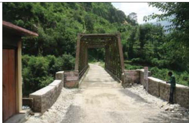
3 Ghansali Tehri Pratapnagar Motor Road,C.H.-1.2
