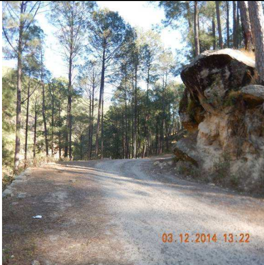
End point of road Bhikiyasain-Deghat-Bungigdhar-Bachuwaban-Mehalchori-Chaukhtutia Motor Road
