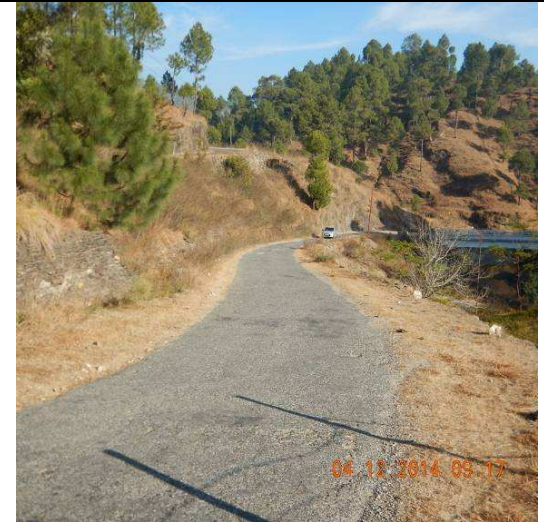
View of road alignment , Kosi-Daulaghat-Binta Motor Road
