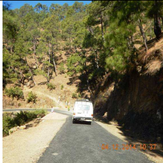
View of road alignment, Kosi-Daulaghat-Binta Motor Road
