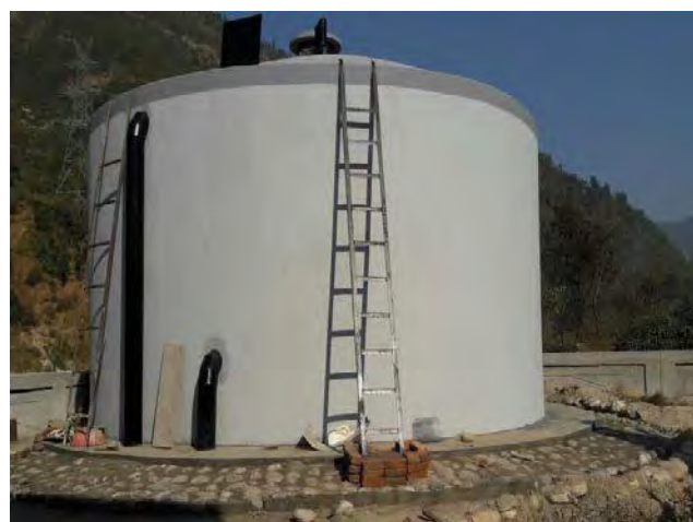
100 KL sump in progress at Kaleshwar, Karanprayag
