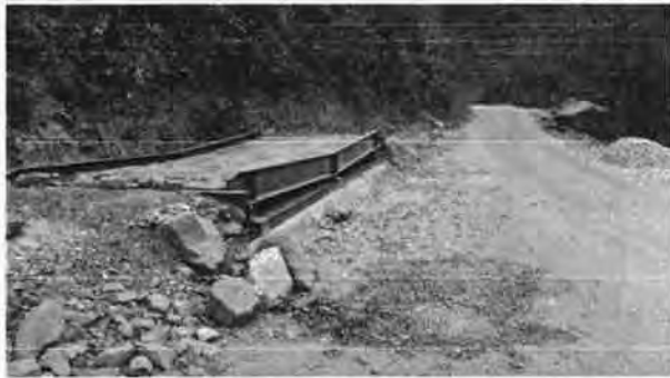
C-29 Weighing machine along road
