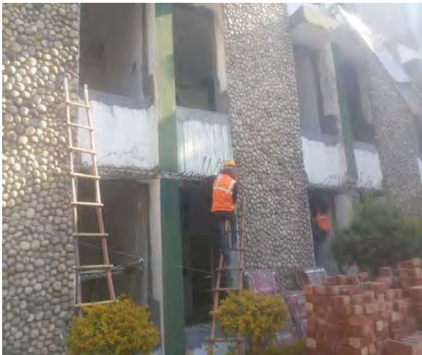
Restoration work at TRH Uttarkashi
