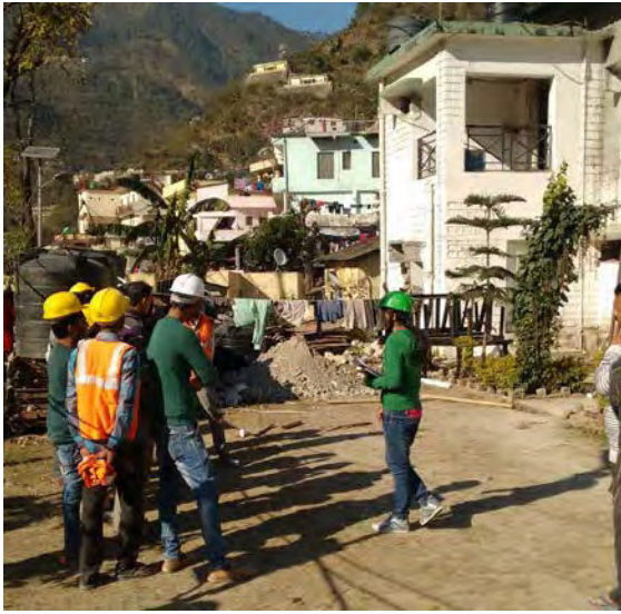
OSHA: Onsite training to labourers
