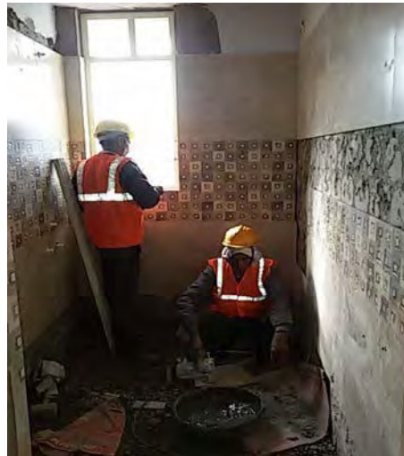
Restoration work at TRH Jakholi
