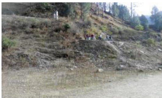
Approach road connect to Mori site
