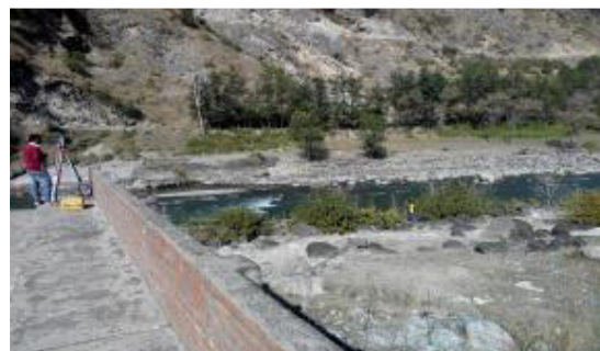
Approach road connect to Tyuni site
