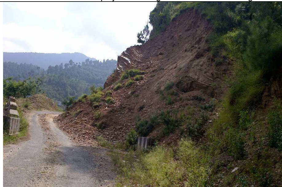
Major slip zone at chainage 15+500 Natuwkhan-Suyalbari Road
