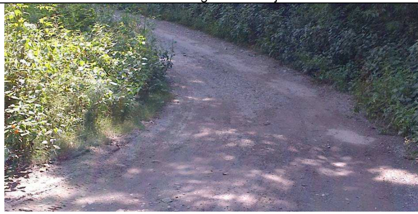
Resurfacing is required near Naugarh Village
