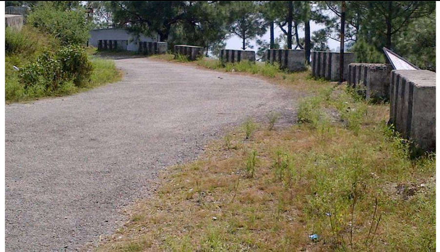
View of project road alignment before meeting to NH-87E, Barely-Almora road
