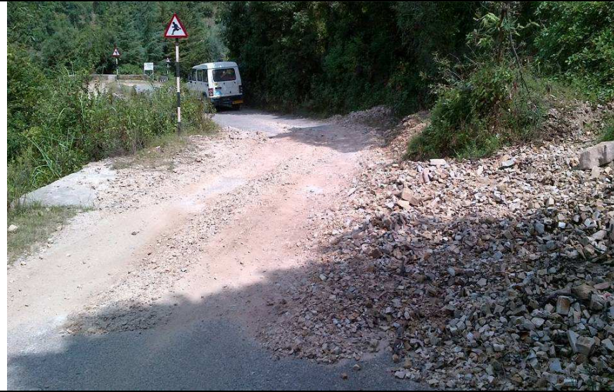
At chainage 0+100 slip zone Natuwkhan-Suyalbari Road
