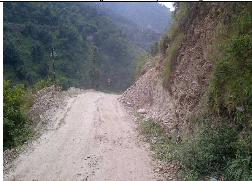
Major slip zone at chainage 15+500 Natuwkhan-Suyalbari Road
