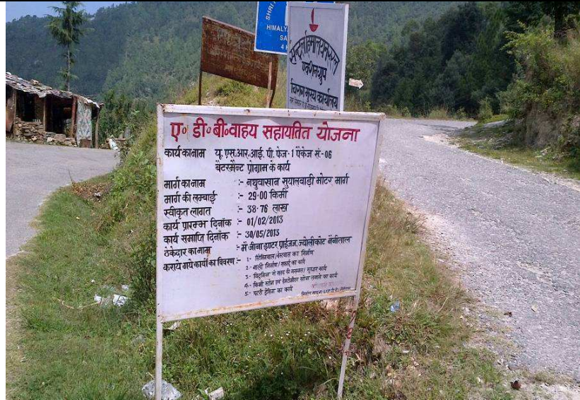
Start point of Nathuwkhan- Suyalbari subproject road
