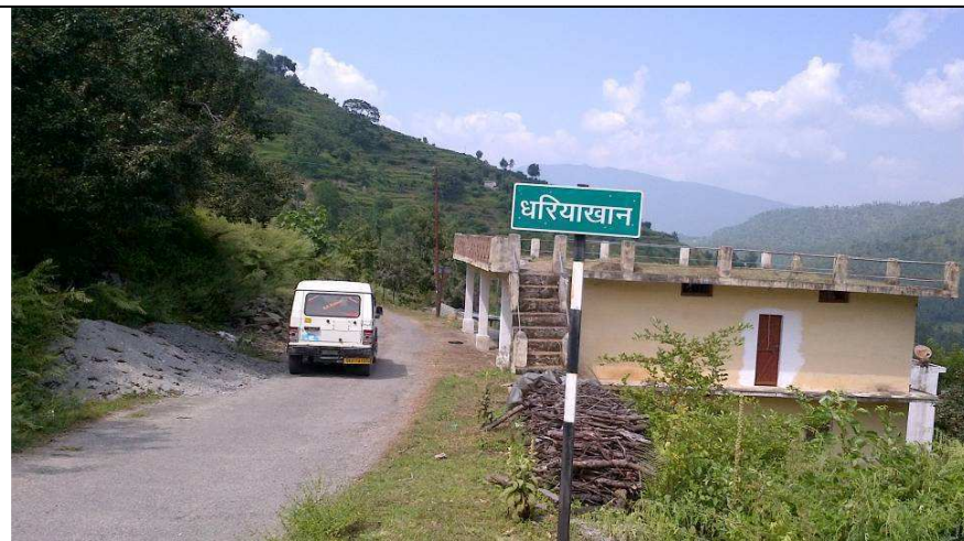
View of road alignment at Dhariyakhan Village
