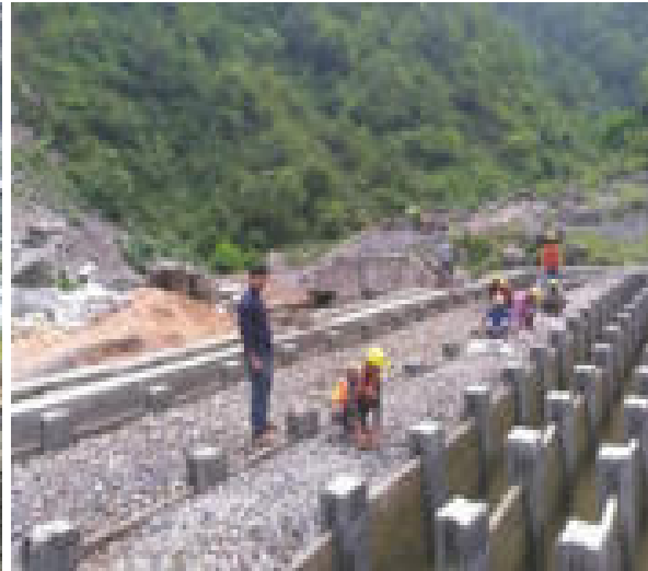
Workers with PPE at Dharchula HRF
