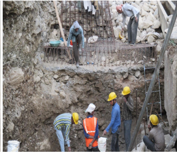
Workers with PPE at Uttarkashi retaining wall
