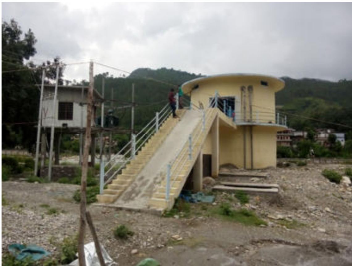
Completed Infiltration well at Kapkot UK/UEAP-UJS/WSS-KU/01/2014-15(Lot 1-Kapkot)
