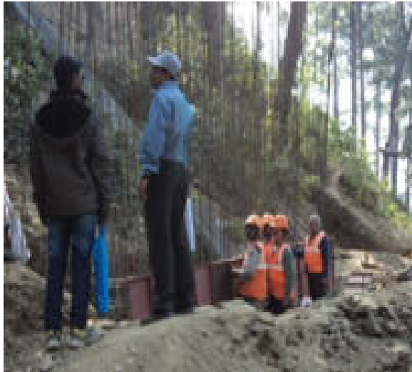
Workers with PPE at Karnaprayag retaining wall
