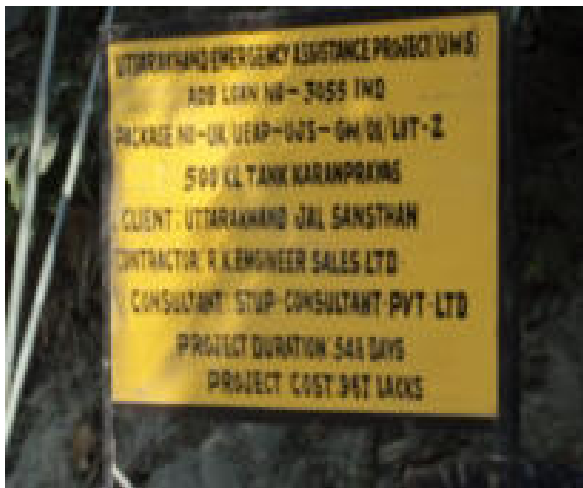
Project signboard at Karnaprayag
