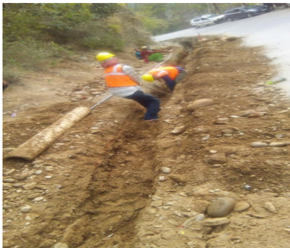
Workers with PPE at Devprayag Pipe laying work
