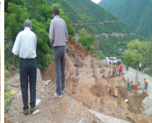
Workers with PPE at Devprayag building site
