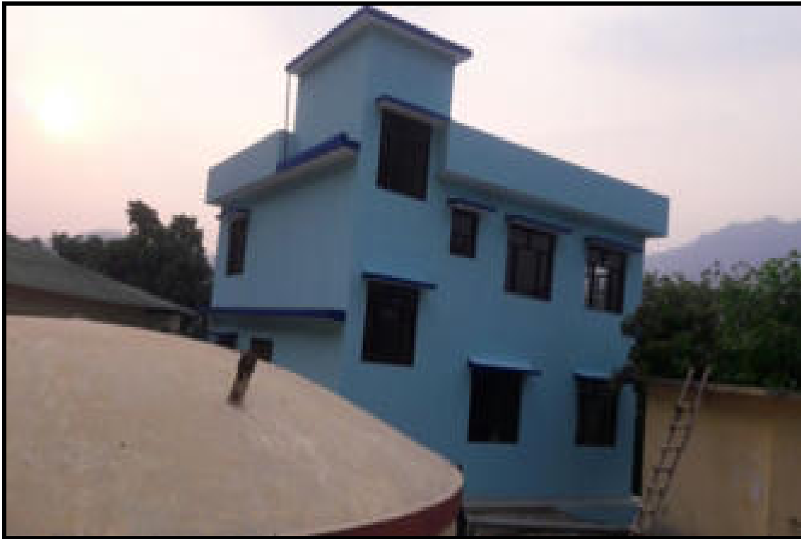
Completed office building at Srinagar (UK/UEAP-UJS/WSS-GW/02-01/SRINAG)
