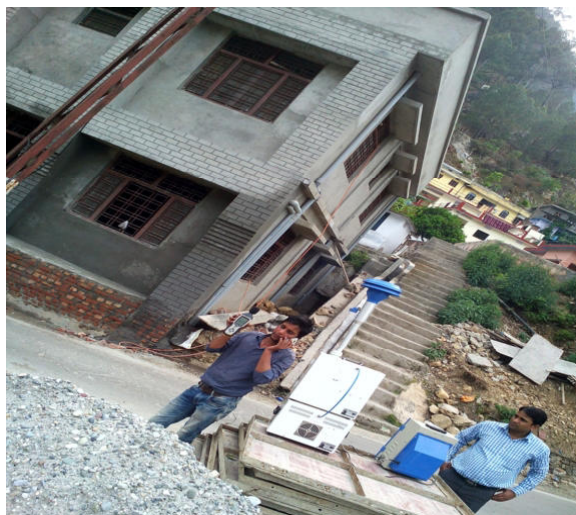
AIR MONITORING AT KARNAPRAYAG
