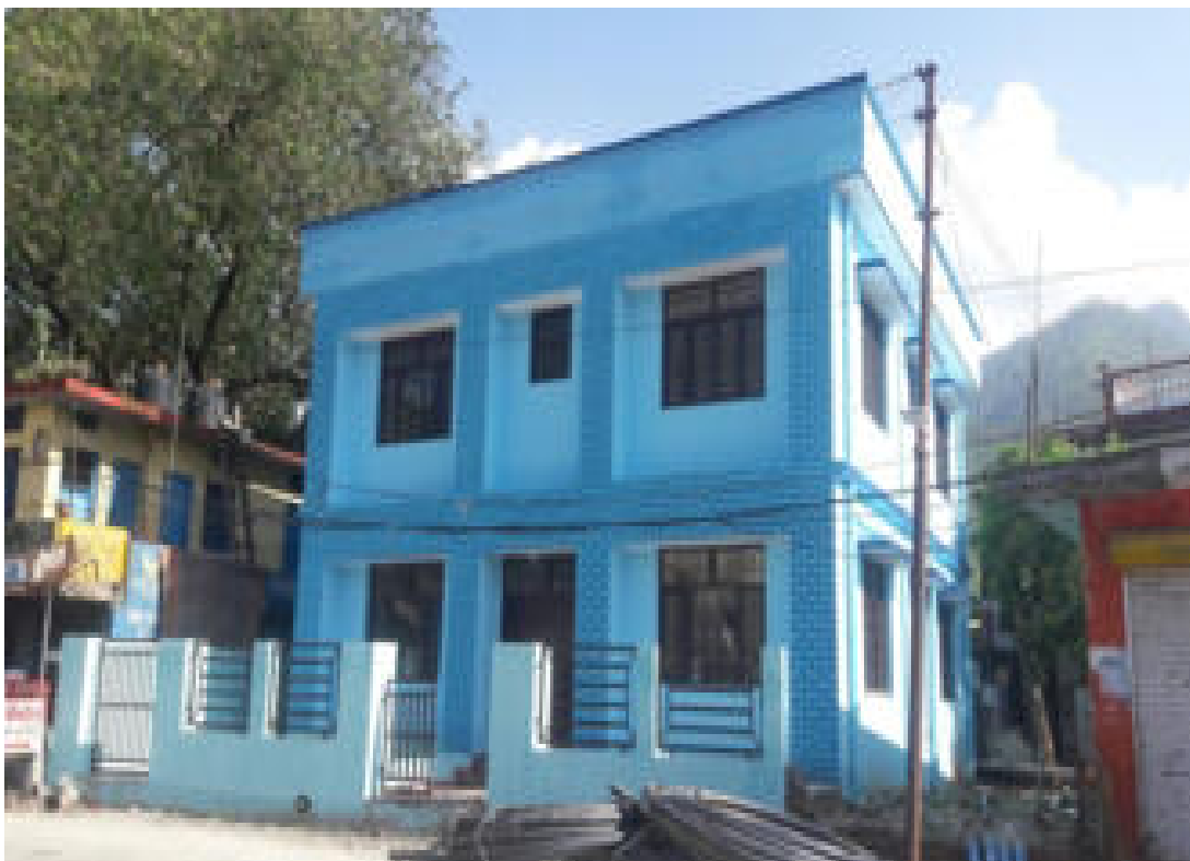
Completed office building at Gauchar UK/UEAP-UJS/WSS-GW/01(Lot 03-Gauchar)
