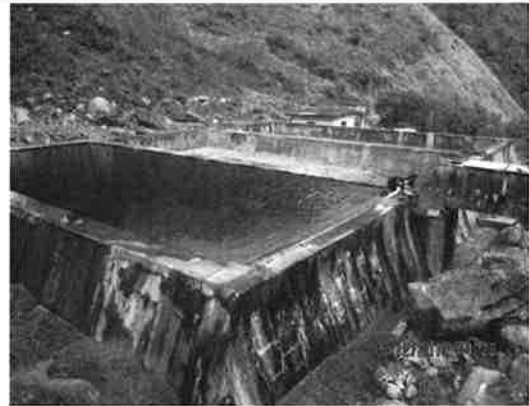
Plate -2- Slow Sand Filter at Galatigarh Gadhera
