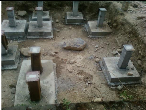
Tilwara: RCC work of column footing
