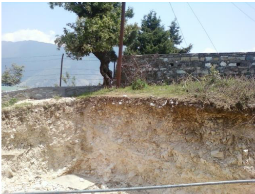
Lohjung: RCC work in column footing is in Progress
