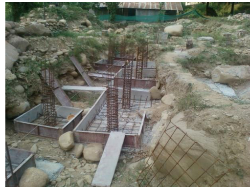
Tilwara: RCC work of column footing
