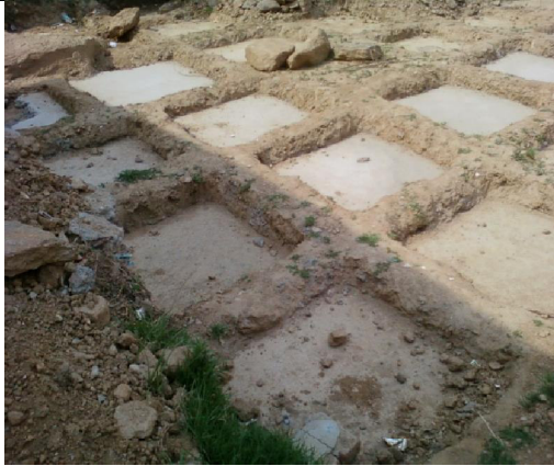
Joshimath: RCC work in Column footing
