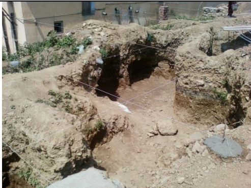
Triyugarayan: Excavation for foundation
