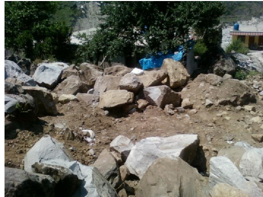
Pandukeshwar: Hill cutting and excavation work for foundation is under progress
