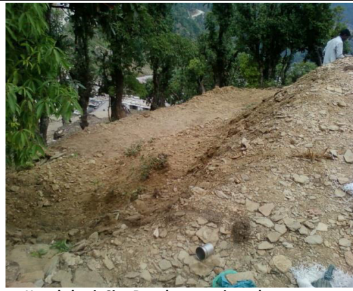
Kanakchori: Site Development is under progress
