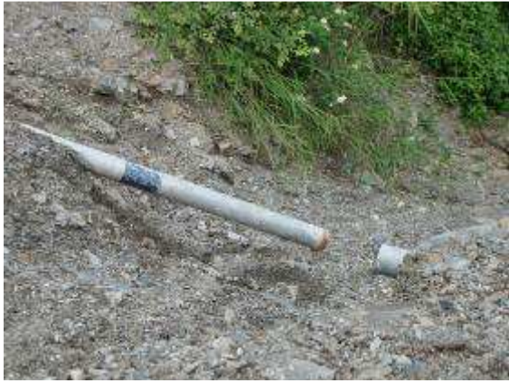
Plate -1-Pipes damaged during the disaster.
