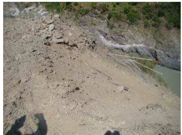
Plate -4-damaged pipes due to disaster
