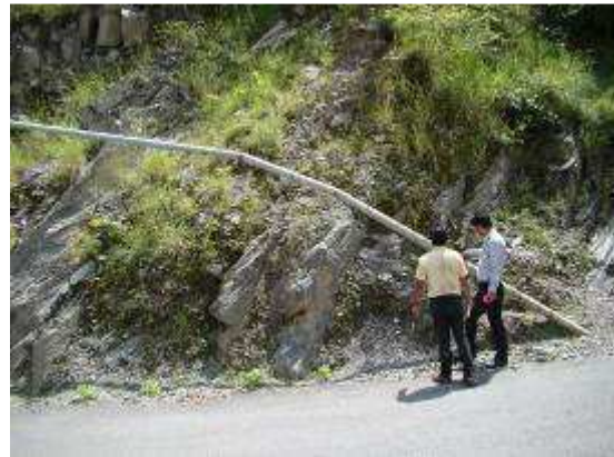
Plate -2- Pipes damaged in Devprayag
