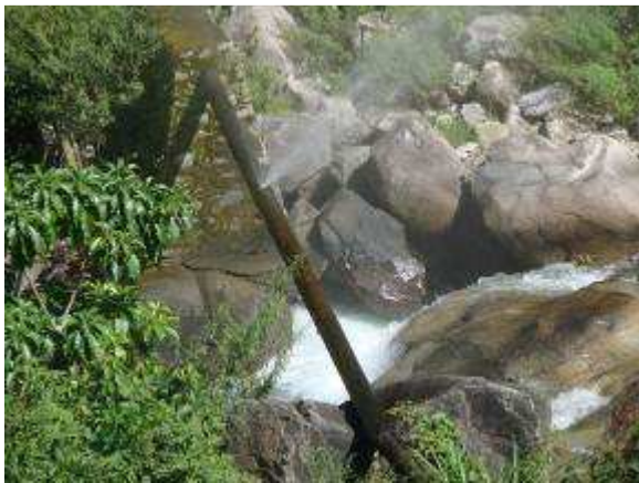
Plate -3- Damages of pipes
