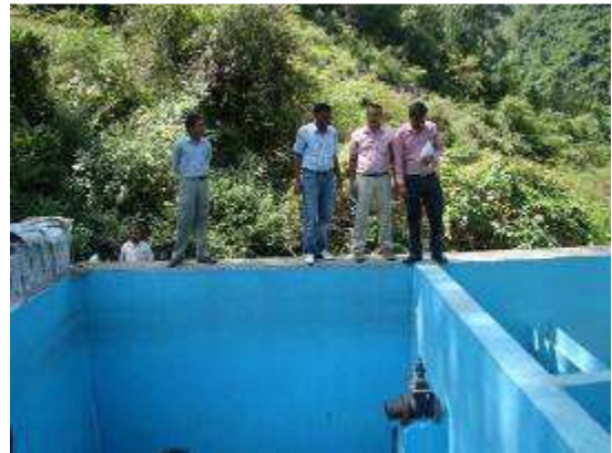
Plate -2- Water Treatment Plant near the source at Sujibagar
