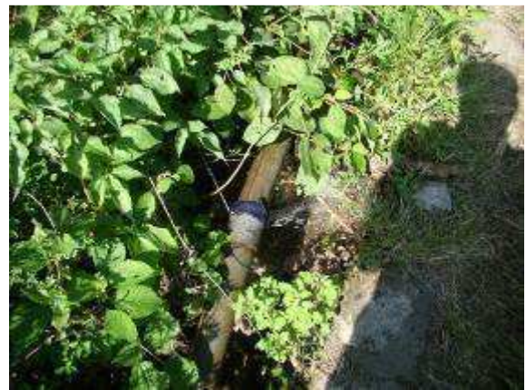
Plate -4-damaged pipes due to disaster
