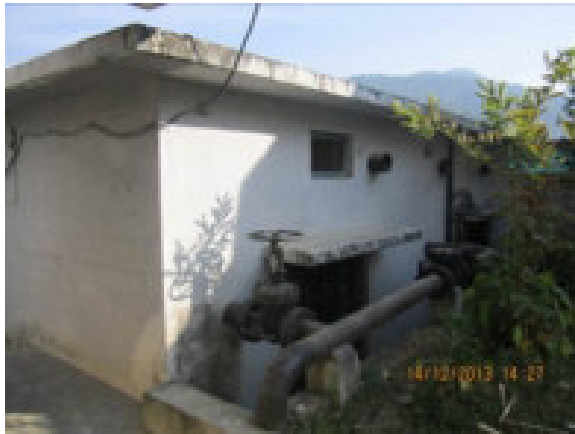
Plate – 9: Clear water Pump house inside Kathyatwada WTP
