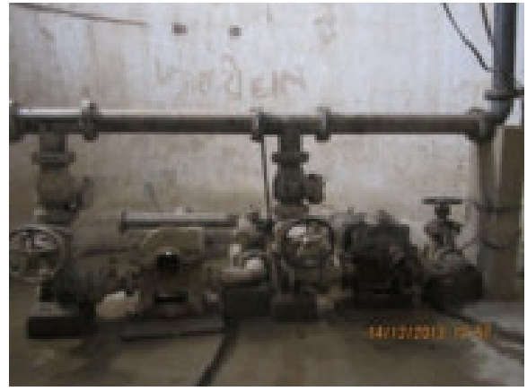
Plate – 8: Dry Intake Well at Kathyatbada- Site where raw water pumps replacement is proposed
