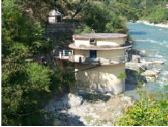
Plate – 7: Dry Intake Well at Kathyatbada
