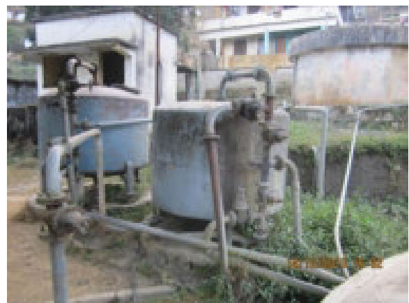
Plate - 12: Old WTP at Thakurdwara – Site where filter media of pressure filters will be replaced
