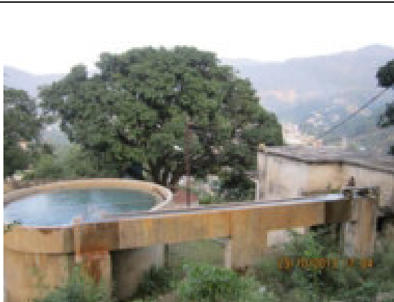
Plate - 11: Old WTP at Thakurdwara – Site where rehabilitation of settlers will be carried out
