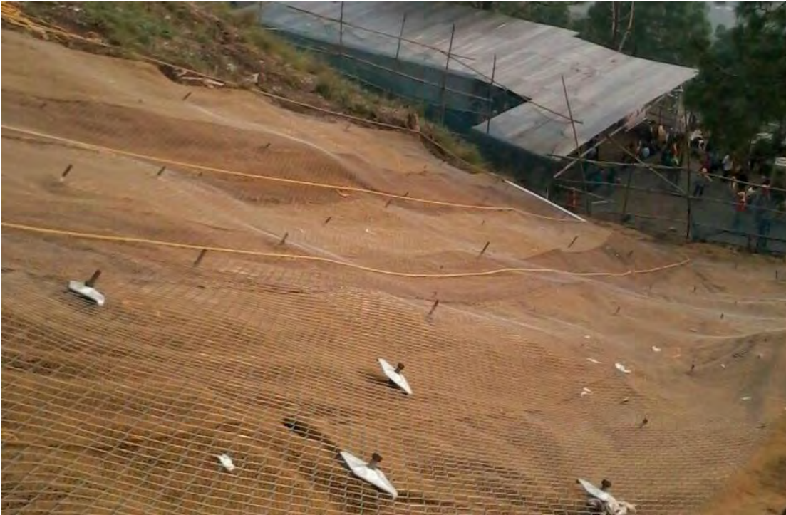
Fig III.4 : View of execution of High Tensile Steel wire Mesh
