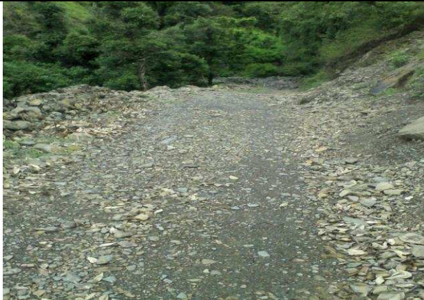
Tehri Ghansali Tilwara Road,C.H.-27.3
