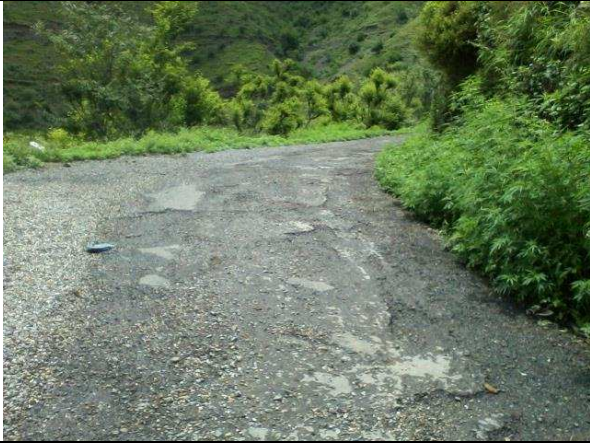
Tehri Ghansali Tilwara Road,C.H.-10.5
