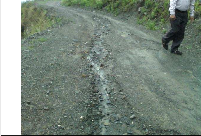
Tehri Ghansali Tilwara Road,C.H.-3.3
