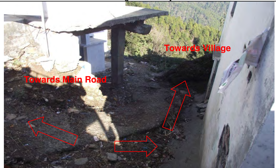
Community asked for construction of approach road which connect Main road near Chorlekh village
