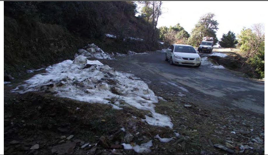
A view of road alignment in Pahadpani area where Snow is observed during site survey
