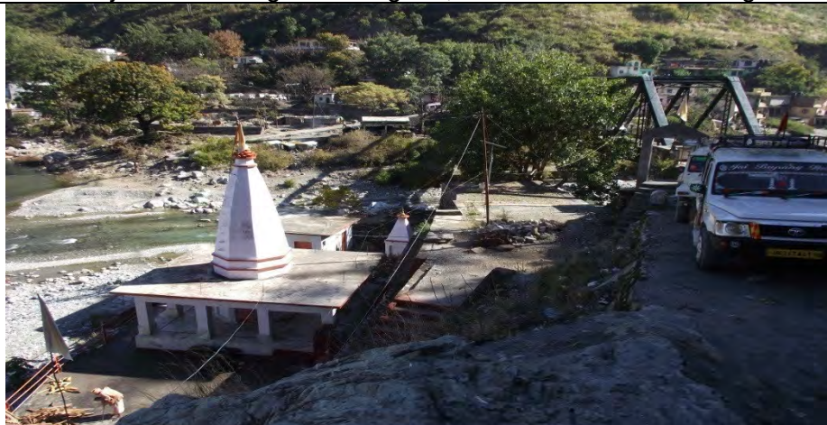
Near Starting point (RHS) there is Temple close to alignment, care should be given during construction
