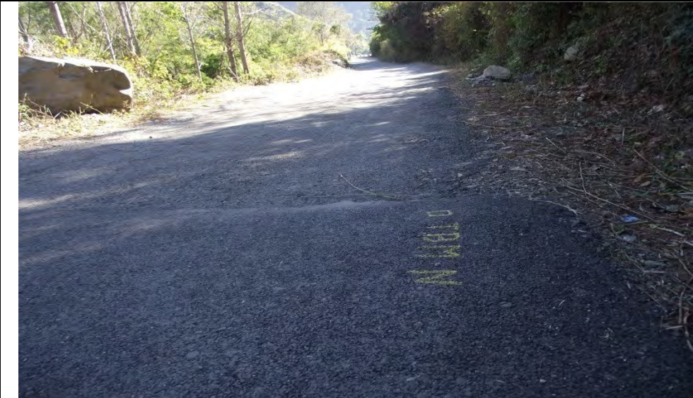
End point of Km 1, after that till km 16 road is good and no restoration work has been proposed
