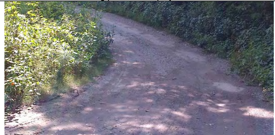
View of road alignment
