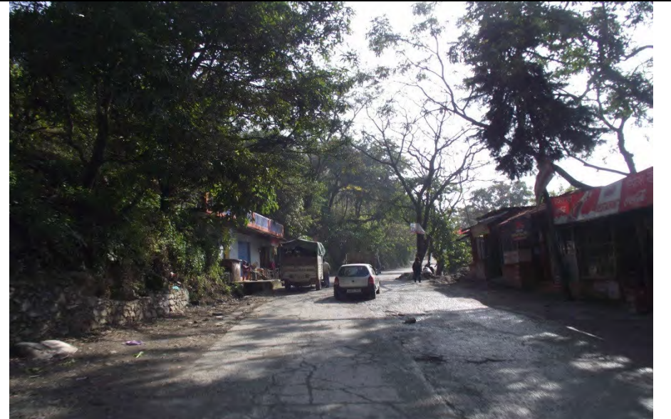
View of road alignment in Km 7 near Saladi village
