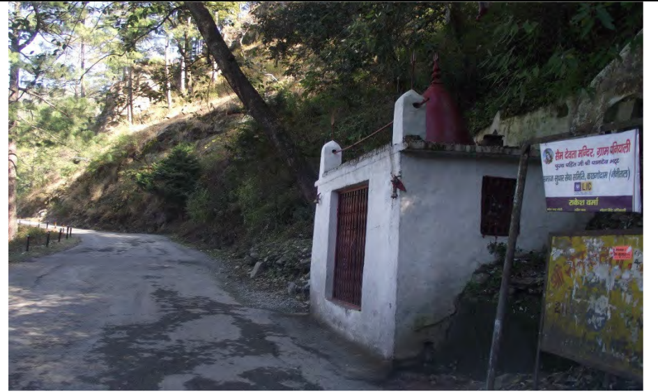
Small religious structure along the alignment , care should be taken during construction.
