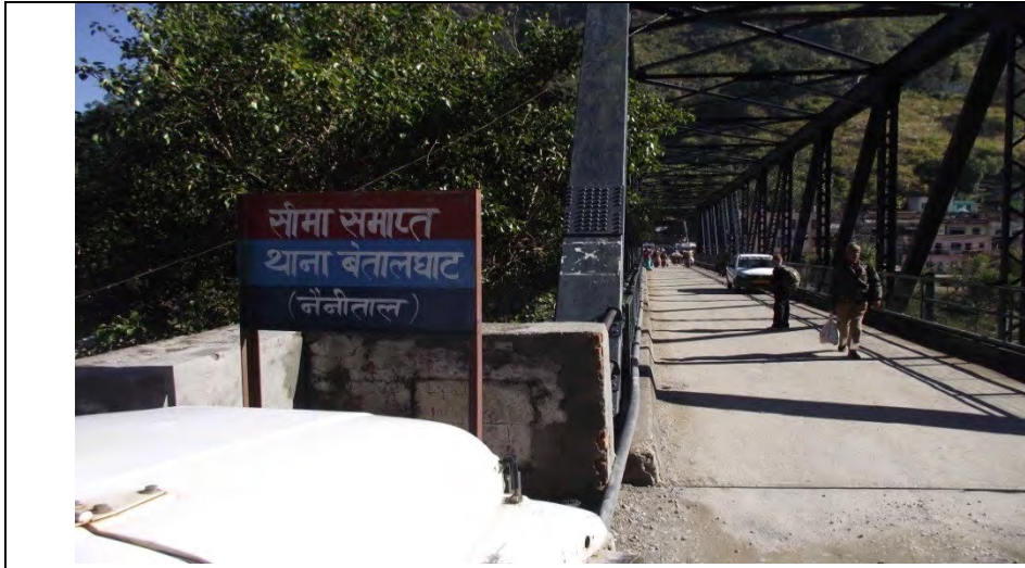
Project road Ratighat-Betalghat , starts Just after this bridge
