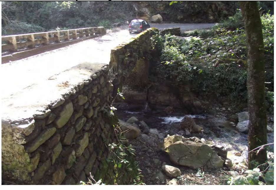
View of Minor bridge at km 23+500 , need to be reconstructed/restored
