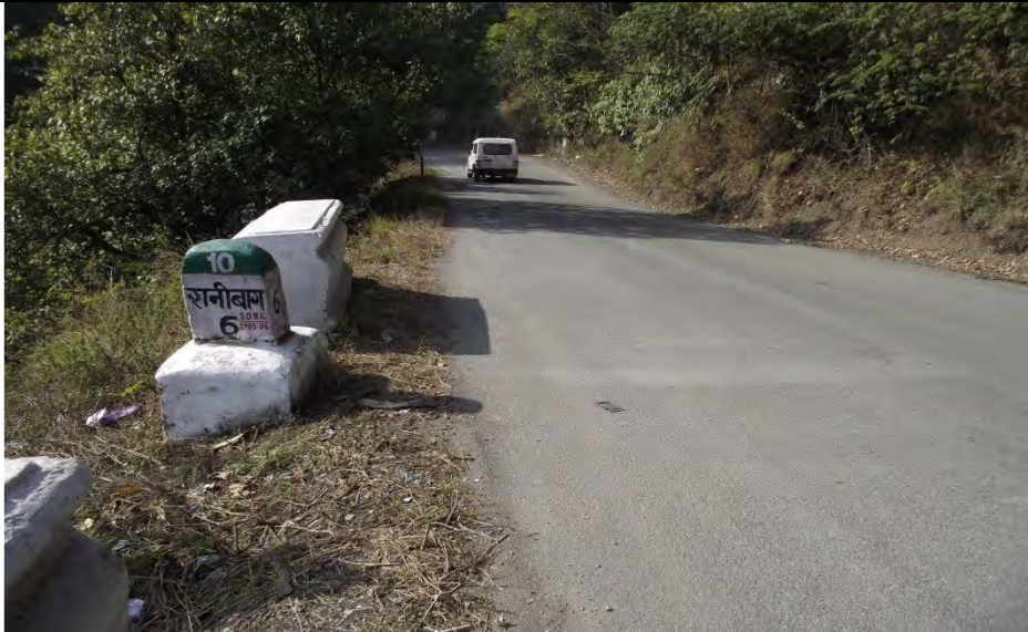
Start point of road RAnibag-Bhimtal-Khutani-Padampuri-Motipathar-Logaghat Motor Road.
