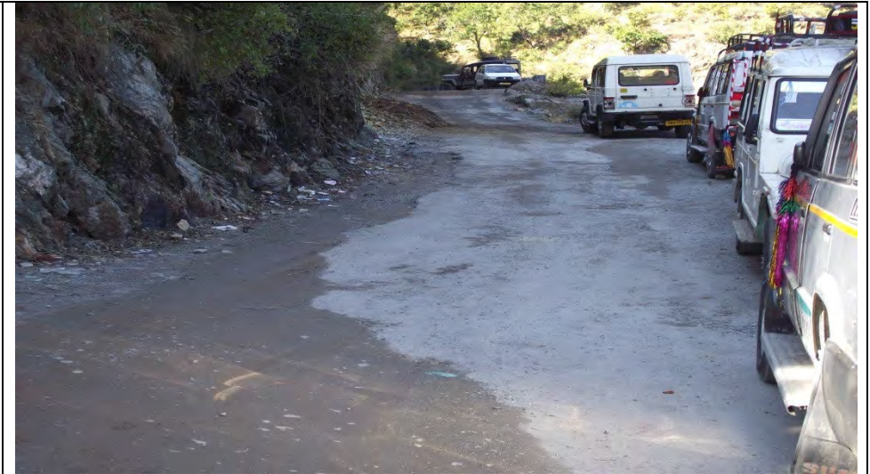
Starting point of Sub-project road
