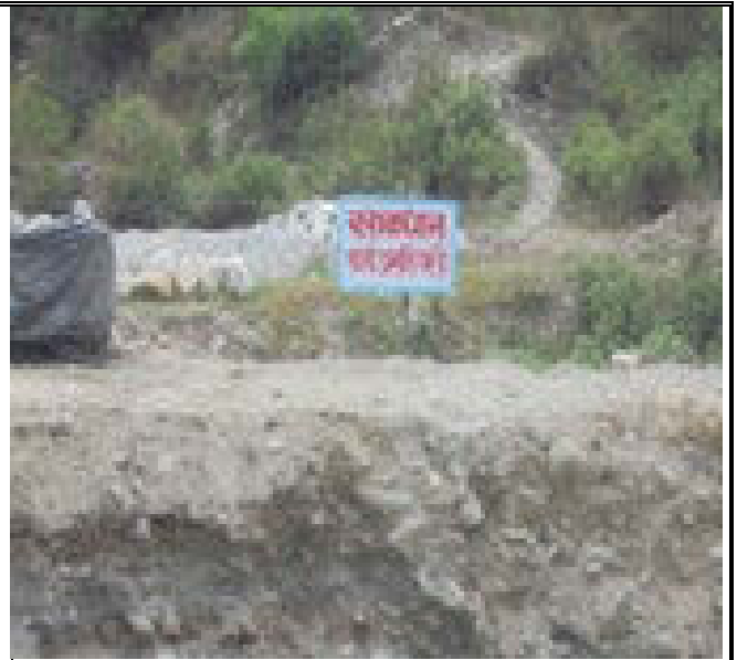
Plate – 2: Danger symbol(s) displayed by the contractor near construction site for alertness (Photograph taken on 1 st June, 2015)
