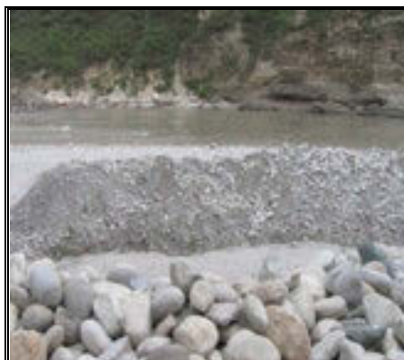
Plate – 17: Excavation work for retaining wall on the Bank of Alaknanda River at Gauchar (Phototaken on 30 May, 2015)
