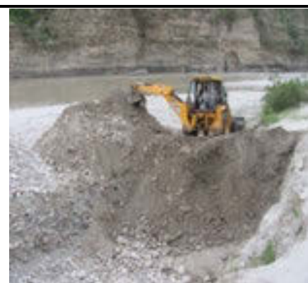
Plate – 18: Excavation for retaining wall, Gauchar (Photograph taken on 30 May, 2015)
