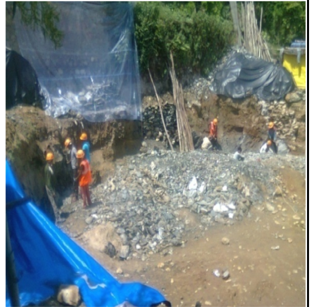
Plate – 24: Excavation for 1000 KI GLSR at Srinagar
