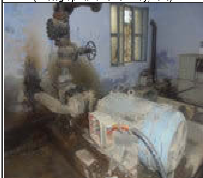
Plate – 7: Damaged Pump to be replaced at Kathayatbada (Photograph taken on 31 st May, 2015)
