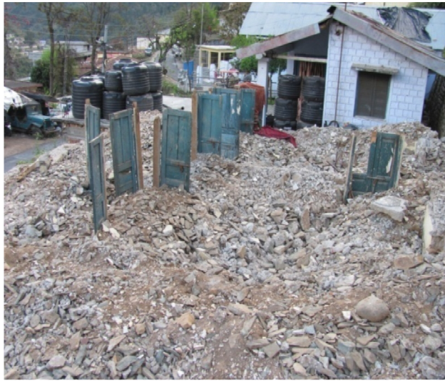
Plate – 13: Office Building Construction work at Karnaprayag (Photograph taken on 30 May, 2015)
