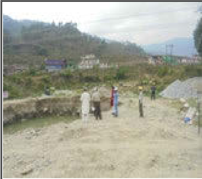
Plate – 1: Infiltration well under construction at Kapkot (Photograph taken on 1 st June, 2015)
