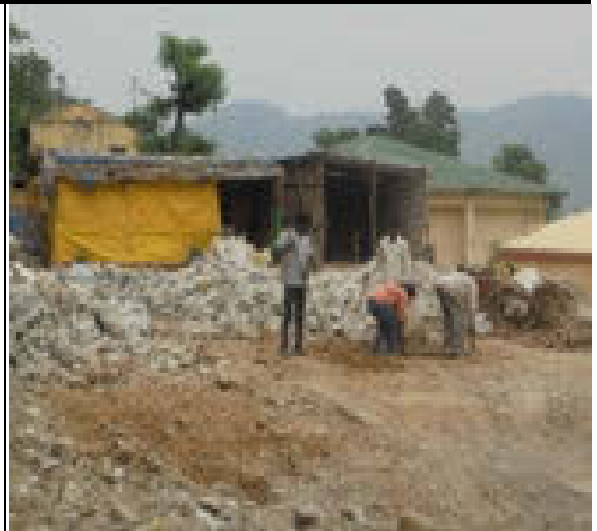
Plate – 22: Excavation Work under progress for 1000 KL near Dangbunglaw at Srinagar
