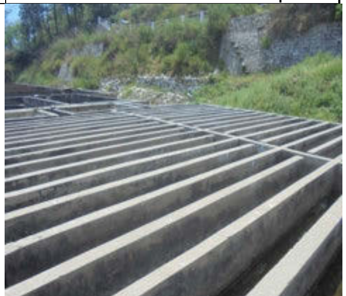
Plate – 32: Water filtration channels at Gofiara, Uttarkashi (Photograph taken on 12 th June, 2015)
