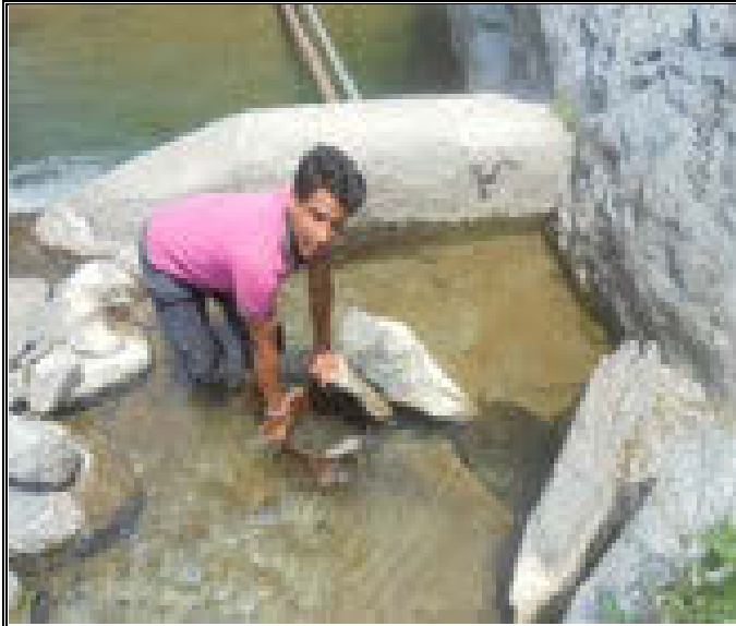
Plate – 25: Existing Intake Well at Source of Randhi Gad near Devprayag (Photograph taken on 29 th May, 2015)
