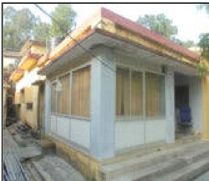
Plate – 19: Existing Office Building to be Renovated (Photograph taken on 30 May, 2015)
