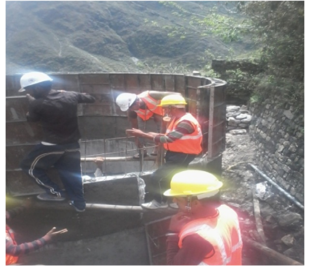
Plate – 10: Tank Construction at Dharchula
