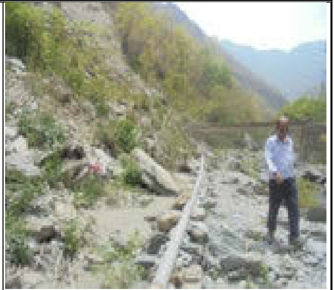
Plate – 26: Damaged Pipe Line due to Landslide at Randhi Gad near Devprayag (Photograph taken on 29 th May, 2015)
