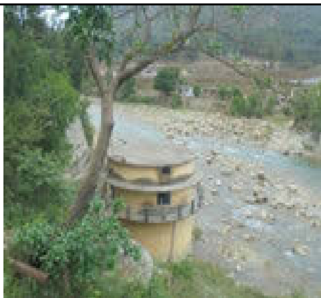
Plate – 6: Damaged pump house at Kathayatbada, Bageshwar (Photograph taken on 31 st May, 2015)
