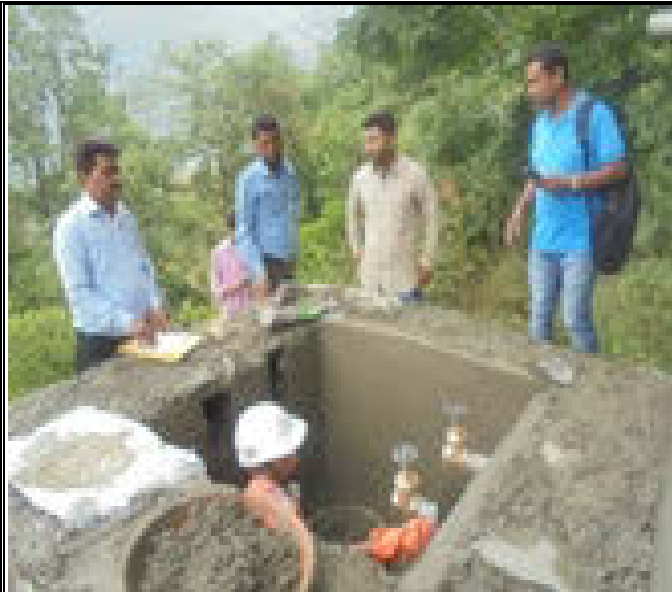
Plate – 9: Construction of Outlet Chamber at Manakhet, Dharchula (Photograph taken on 2 nd June, 2015)
