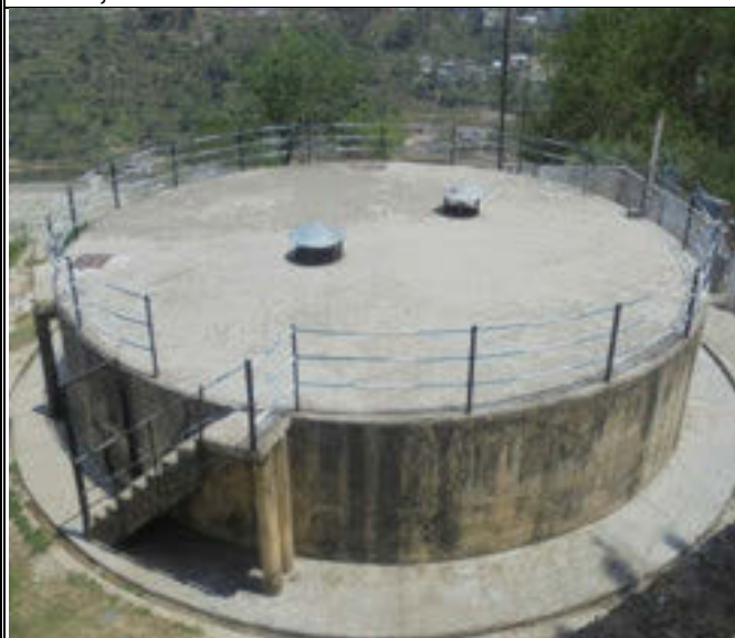
Plate – 31: Existing water tank at Gofiara site for minor repair work Photograph taken on 12 th June, 2015
