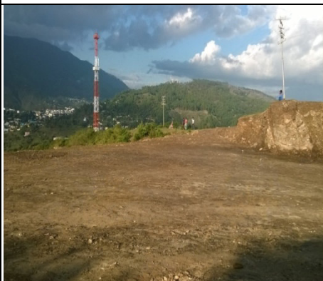
Plate – 13: Excavation work at Dwarahat helipad site (View - I)
