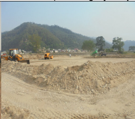
Plate – 11: Excavation work at Chaukhutia helipad site (View-II)
