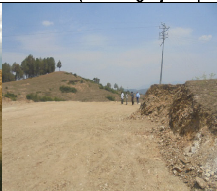
Plate – 14: Excavation work at Dwarahat helipad site (View - II)
