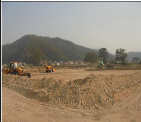
Plate – 10: Excavation work at Chaukhutia helipad site (View - I)
