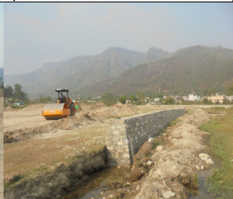
Plate – 12: Construction of retaining wall at Chaukhutia site
