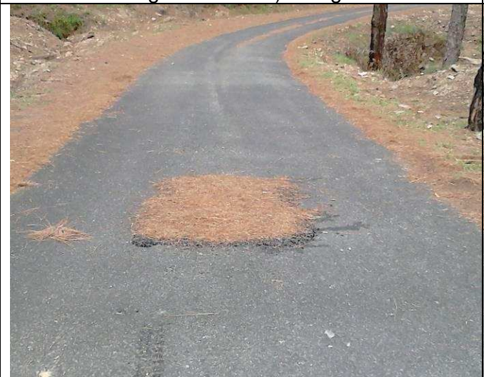
Repairing work is being carried out under USSRP (Jalikhan-Nobara road )
