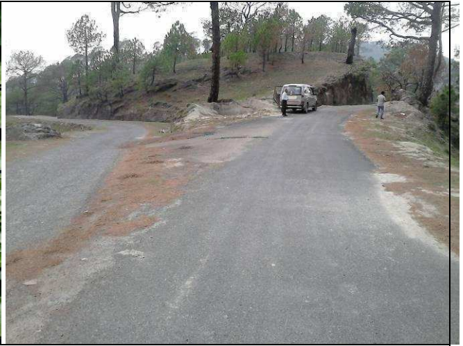
Start point of road Jalikhan-Nobara –no habitation
