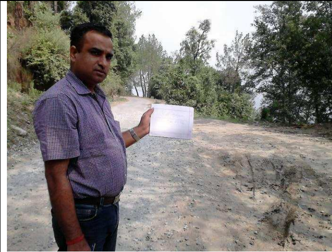
At chainage 19+900 damaged road ( Almora-Bageshwar)
