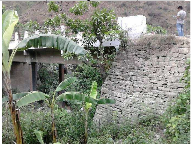
RCC single span bridge to be reconstructed parallel to existing bridge ((Almora-Bageshwar road)- village Pilaona.
