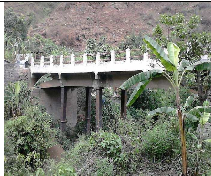
Existing RCC single span bridge (Almora-Bageshwar road)- village Pilaona.
