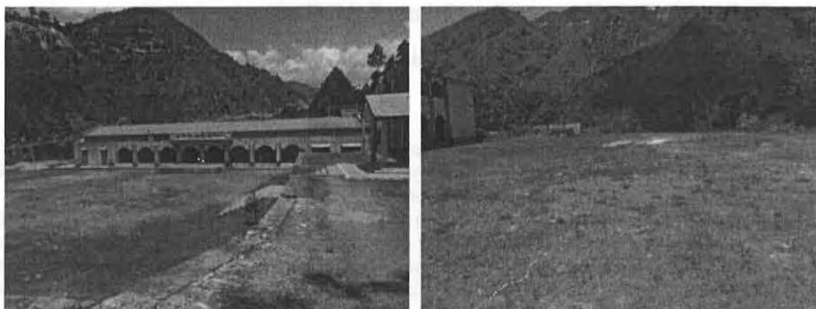
Plate 2: Proposed location for construction of Helipad at Lambgaon
