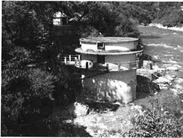
Plate-7 Dry Intake Well at Kathyatbada
