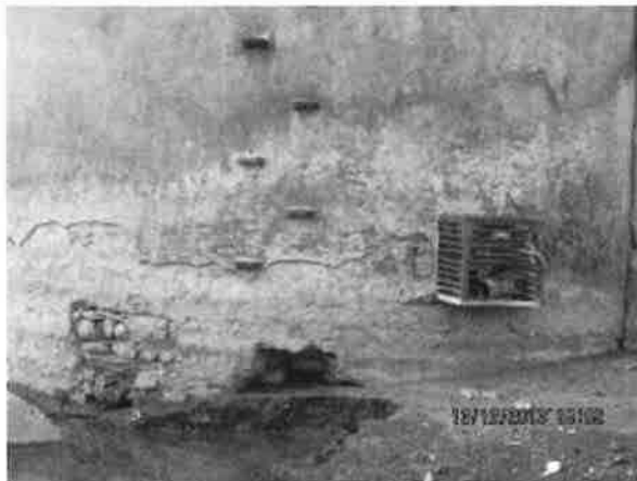
Plate-5 River water level below intake opening at Jalkal Intake Well
