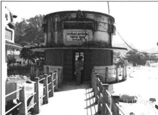
Plate-1 Jalkal Intake Well -Construction Year 1975: Will be demolished and Infiltration well will be constructed in its place
