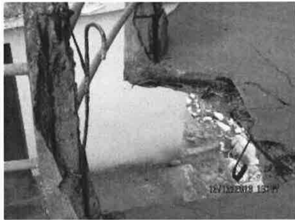
Plate-4 Damaged Cantilever slab in Jalkal Intake Well
