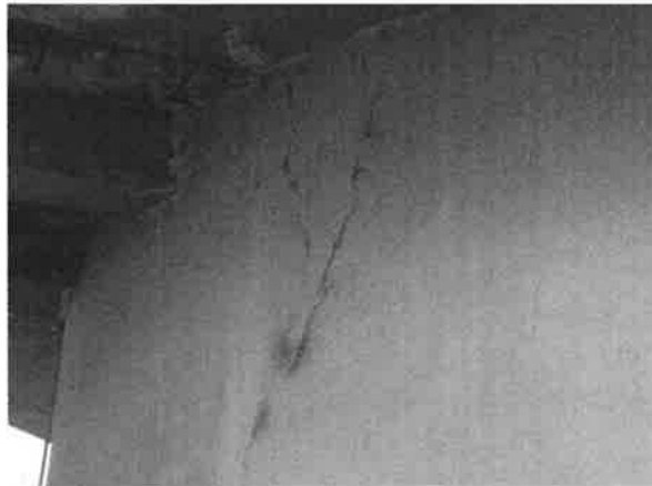
Plate-3 Cracks in Jalkal Intake well
