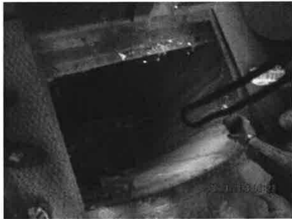
Plate-2 Garbage and silt deposition at Jalkal Intake Well
