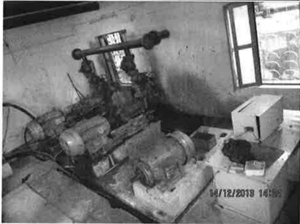
Plate-10 Clear water Pump house inside Kathyatwada WTP - Site where clear water pumps replacement is proposed
