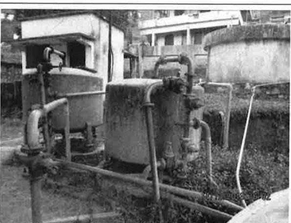
Plate-12 Old WTP at Thakurdwara - Site where filter media of pressure filters will be replaced
