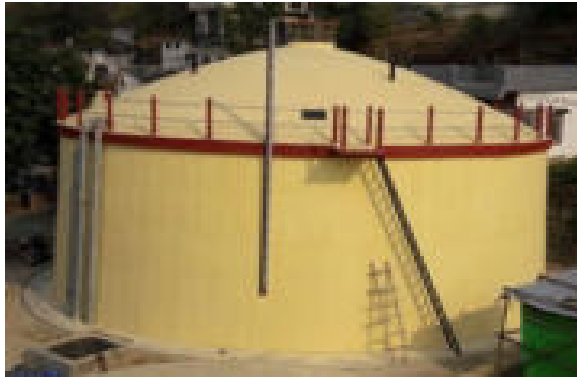
1000KL Water Tank
