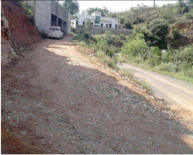
Subproject road alignment of Jaji approach road section- Bageshwar
