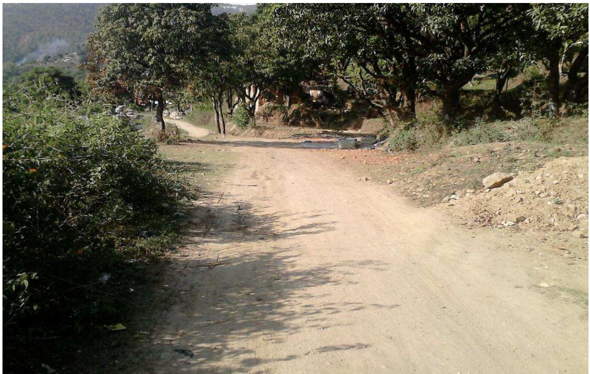
View of subproject section- Ring road –Mandal Sera Section- Bageshwar
