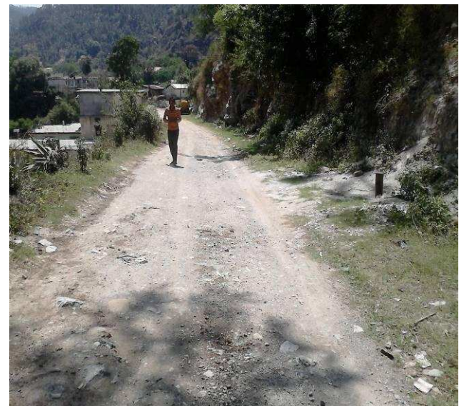
View of subproject road section Bhayun- Gulair
