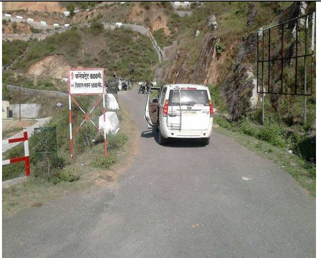
Subproject road section Collectorate approach road - Bageshwar
