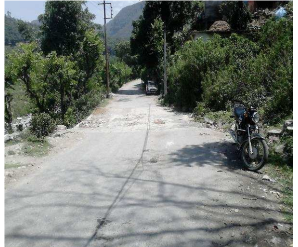
View of subproject road alignment of Kapkot- Karmi section
