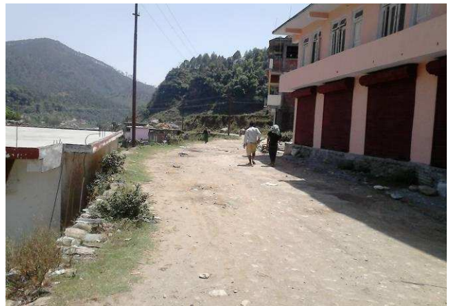
View of subproject road Kapkot- Poling- kapkot Block
