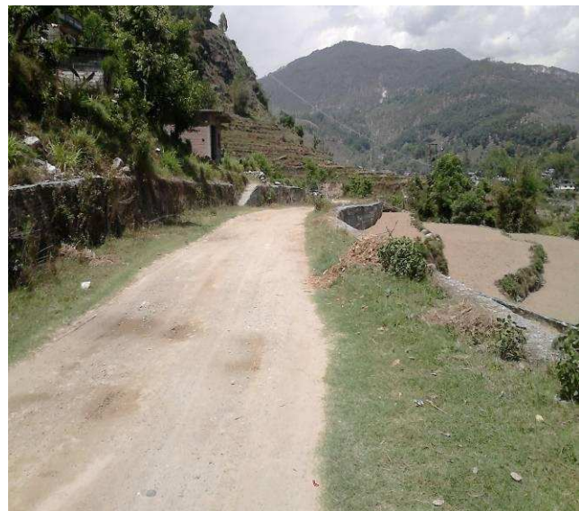
View of subproject road Kapkot- Poling- kapkot Block
