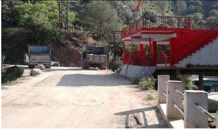
A Hanuman je Temple along subproject road alignment- Ring Road –Mandal Sera section - Bageshwar
