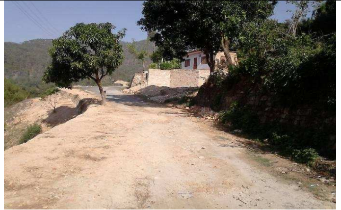
Subproject road section – Pulled house approach road- Bageshwar
