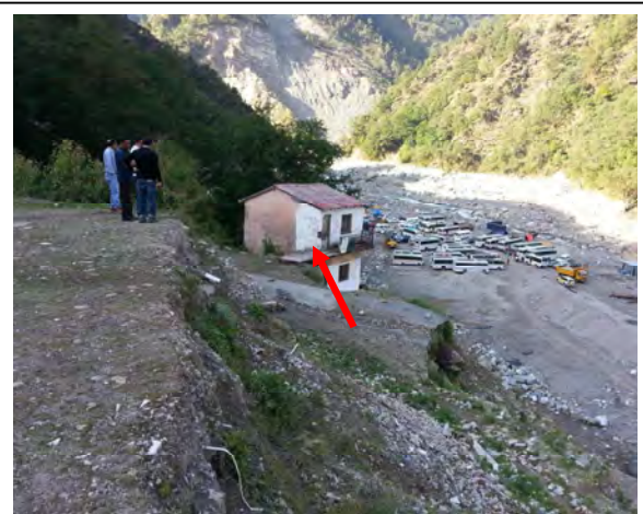
Plate 4: Damaged Tourism Asset at Sonprayag
