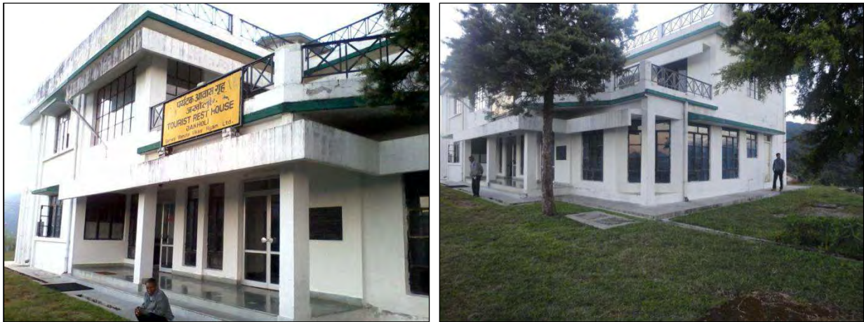
Proposed location for construction of LGFS at Jakholi
