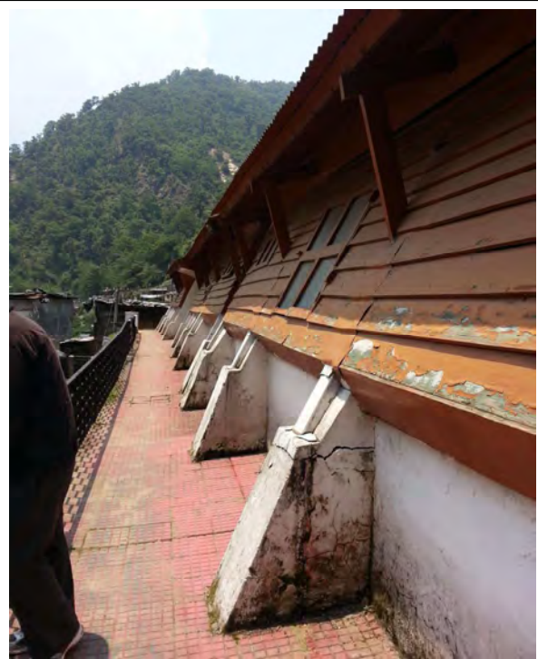
Plate 2: Damaged Tourism Asset Gaurikund
