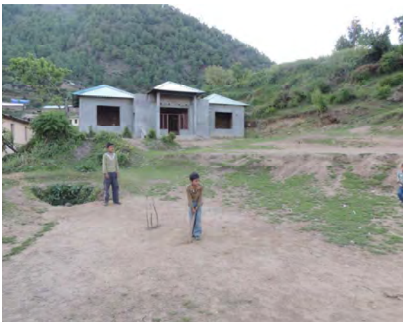
Plate 7: Site for construction of LGFS units at Triyugarayan
