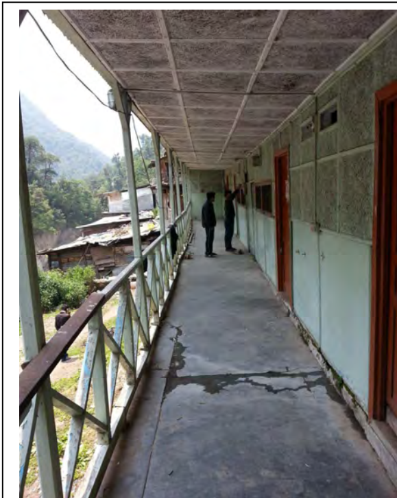
Plate 1: Damaged Tourism Asset Gaurikund
