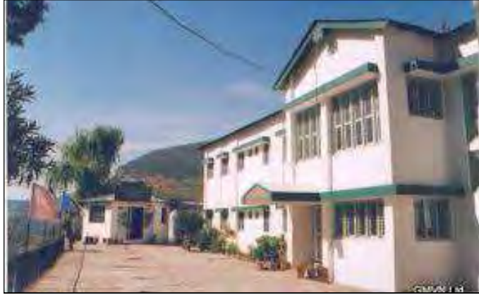
Proposed location for construction of LGFS at Guptkashi
