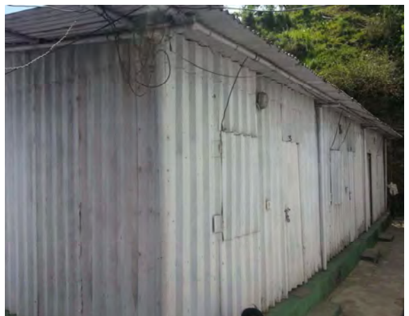
Plate 8: Site for construction of LGFS units at Guptkashi
