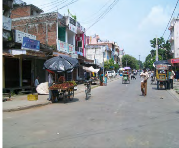
Pilibhit Chungi to Inspection House Metal Roads
