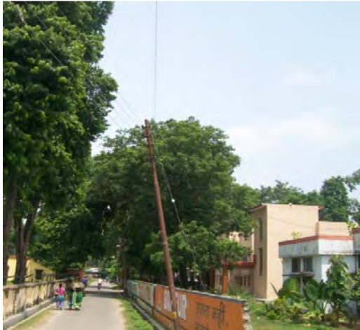
Post Office Metal Road
