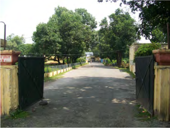
Store Internal Metal Roads
