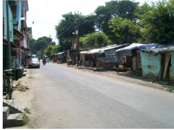
Road side structures at Tanakpur Verma Lane
