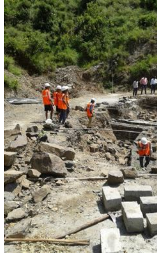
Safety measures at work site, Damta – Kandari road, C-54
