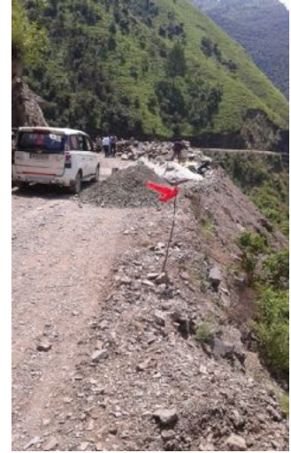
Safety measures at work site Nogaon – Ponty – Rajgad road, C-54
