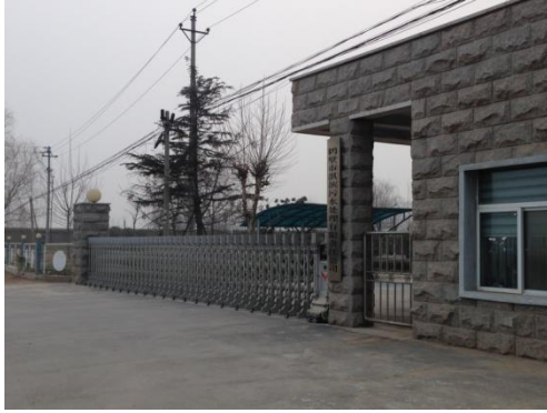
Qibin District WWTP
