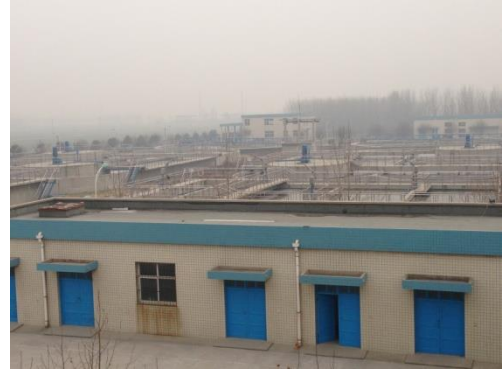
Existing Qi County WWTP
