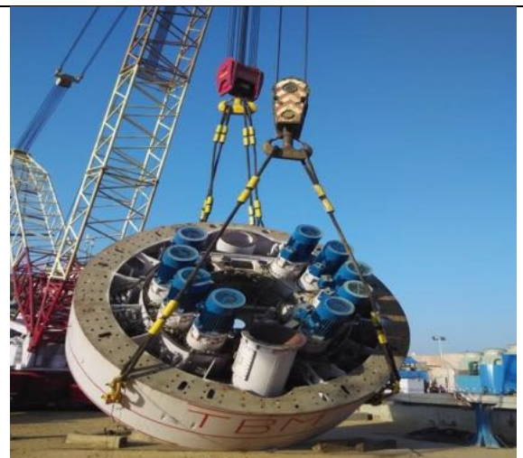
Tilting of TBM-2 at Chandpole Launching Shalft
