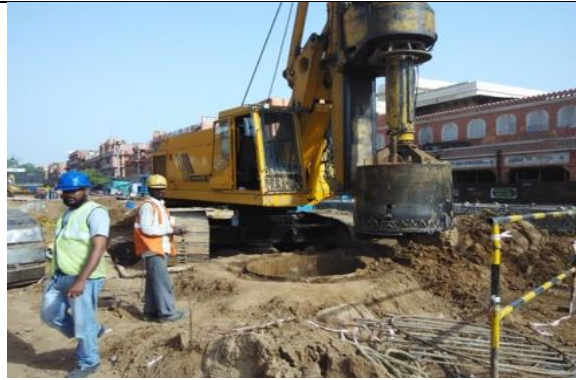
French Collum Excavation at Chhoti Chaupar
