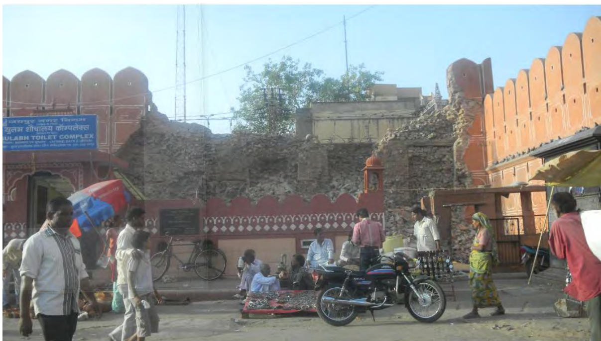
Figure 22: Monsoon Rain Damaged Section of the Wall near Chandpole Gate Showing the Use of Brick and Mud Construction Materials
