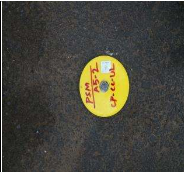
Pavement Settlement Marker
