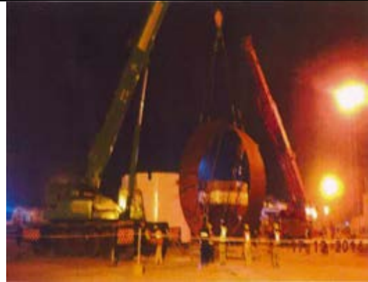
Tilting of TBM-1 Tail Shield
