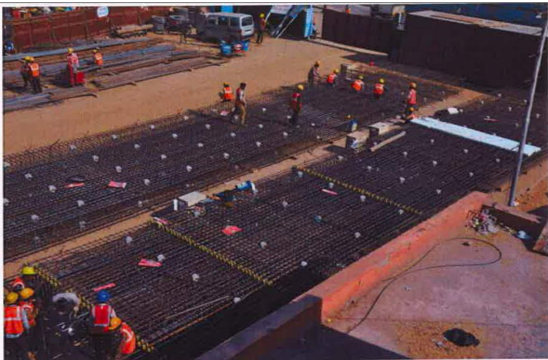
D-Wall Cage Febrication at Chhoti Chaupar
