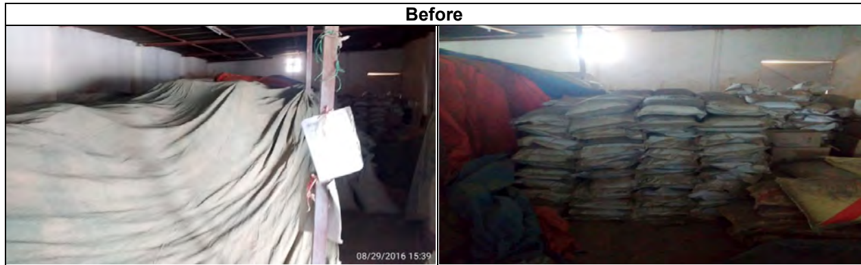
Figures 5 and 6: Improper stacking and segregation of cement bags in the storeroom.
