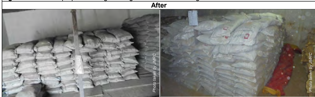
Figures 7 and 8: A system was put in place to stack cement bags according to type with sufficient clearance for convenient access and retrieval.
