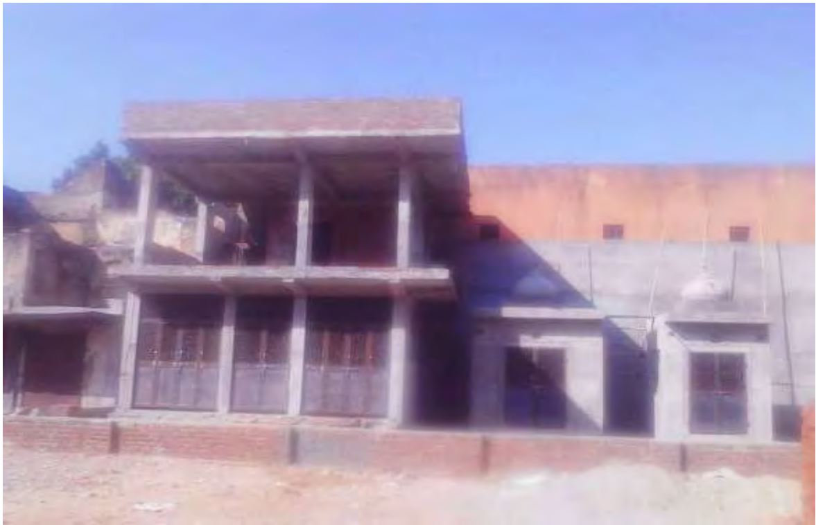
Ongoing construction work at Tanwarji Ka Nauhra (Badi Chaupar Temple Shifting)
