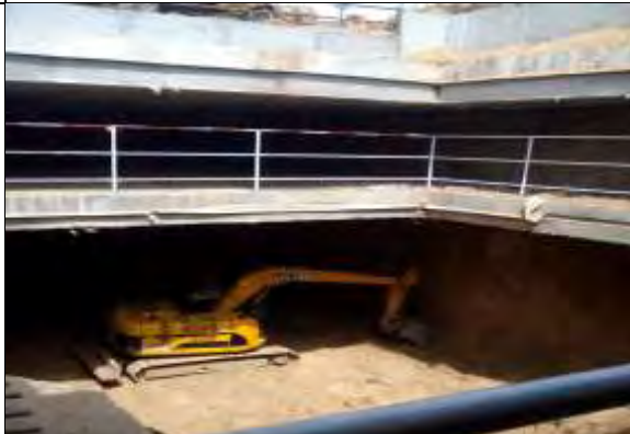
Soil Excavation for Top slab at Chhoti Chaupar
