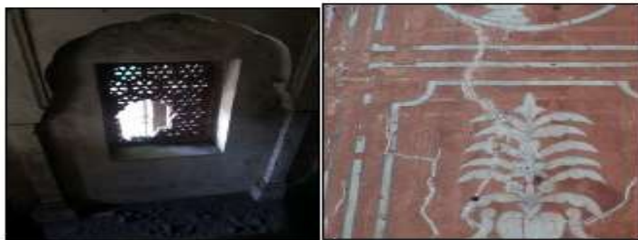
Broken RCC grill, Cracks are being monitored with glass strip to assess widening of cracks
