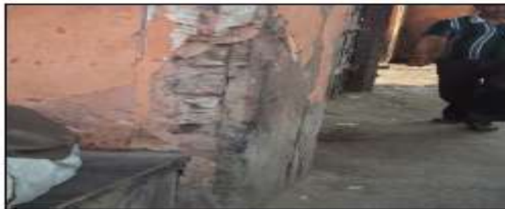
Plaster damaged and stones are exposed.
