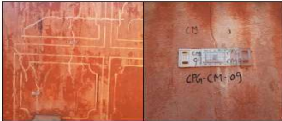
Previous cracks which are being monitored with Crack meters
