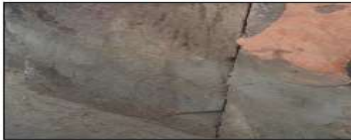
Separation gap/crack is observed between wall and column.
