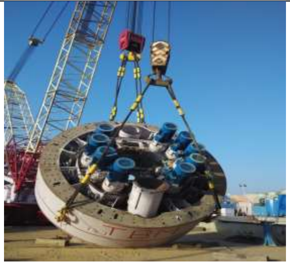
Tilting of TBM-2 at Chandpole Launching Shaft
