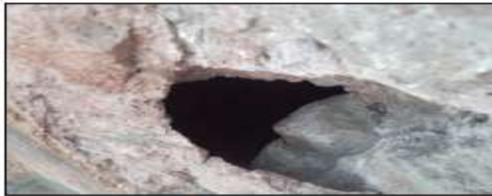
Cavity is observed on wall.
