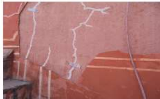
Older plaster cracks on the terrace walls already being monitored. Some of which have marginally expanded but all within permissible limit.
