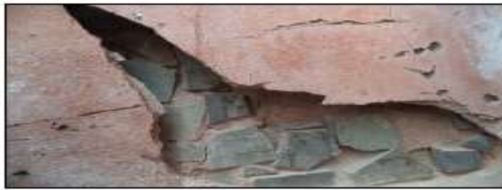
Wall plaster is observed and stones are exposed.
