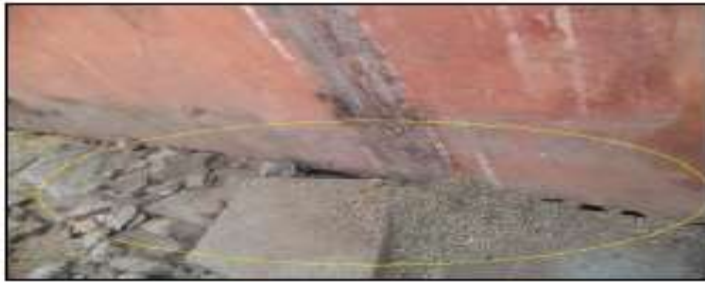
Cavities are formed at wall-ground joint.
