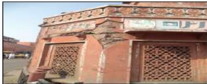
Wall Plaster damaged and stones are exposed.
