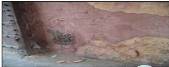
Wall plaster damaged and stones are exposed.
