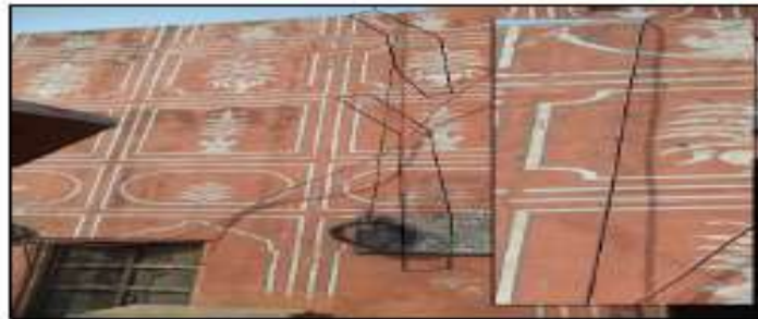
Vertical/ inclined crack is observed on wall.
