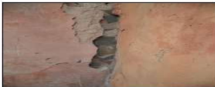
Wall plaster is observed and stones are exposed.
