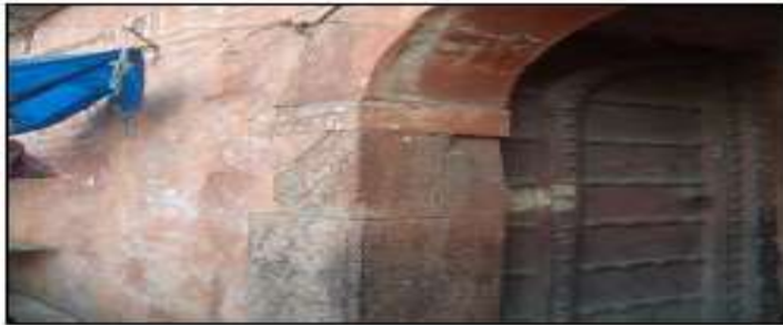
Column plaster damaged and gap is observed between stones
