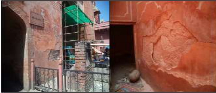
External Plaster damaged and stones are exposed, Internal plaster peeled off near staircase
