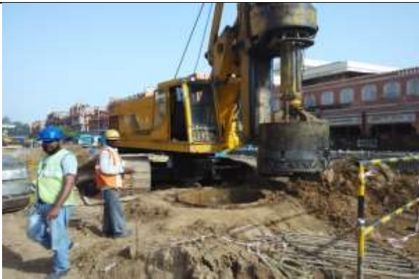
French Collum Excavation at Chhoti Chaupar
