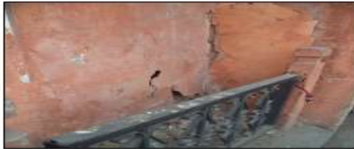
Wall plaster is observed and stones are exposed.
