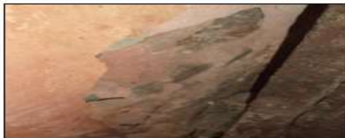
Wall plaster damaged and stones are exposed near gate door.
