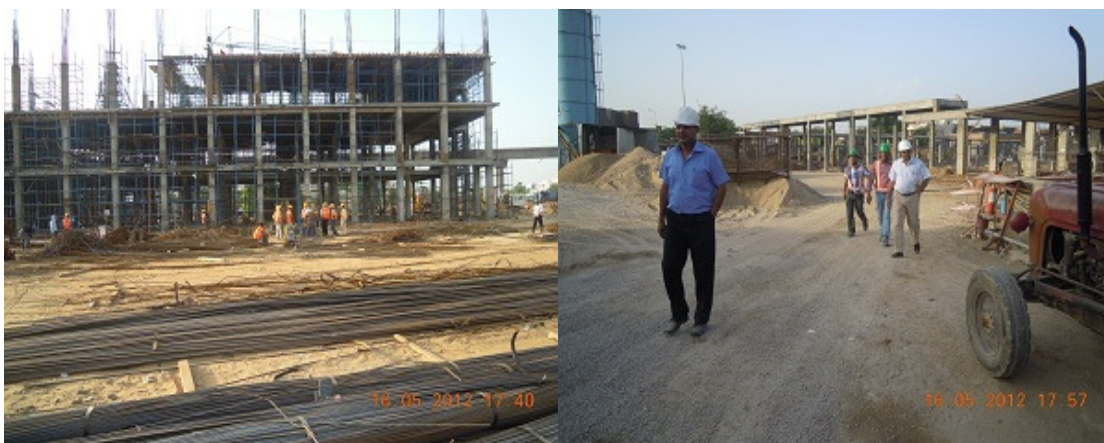
Figure 29: Ongoing Constructions at Mansarovar Depot
