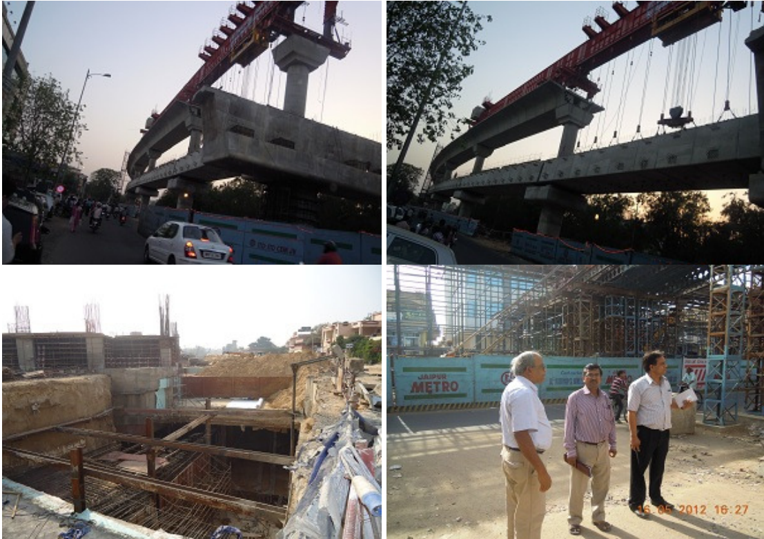
Figure 31: Ongoing construction in Corridor Phase I with safety precautions
