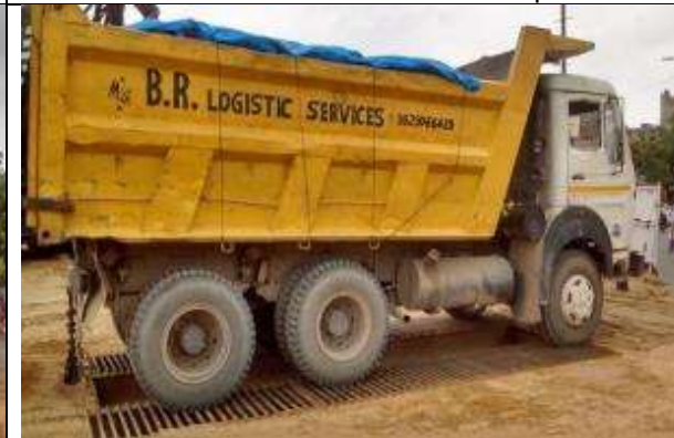
For cleaning the tyre on wheel wash station
