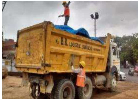
Workers are covering loded dumper with the tarpaulin.
