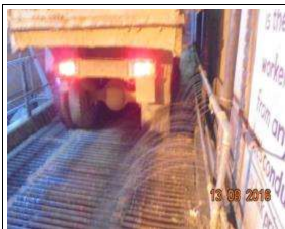
Cleaning the tyre of Loaded dumper before entering the public road.
