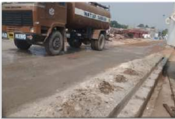
Water Sprinkling through Tank
