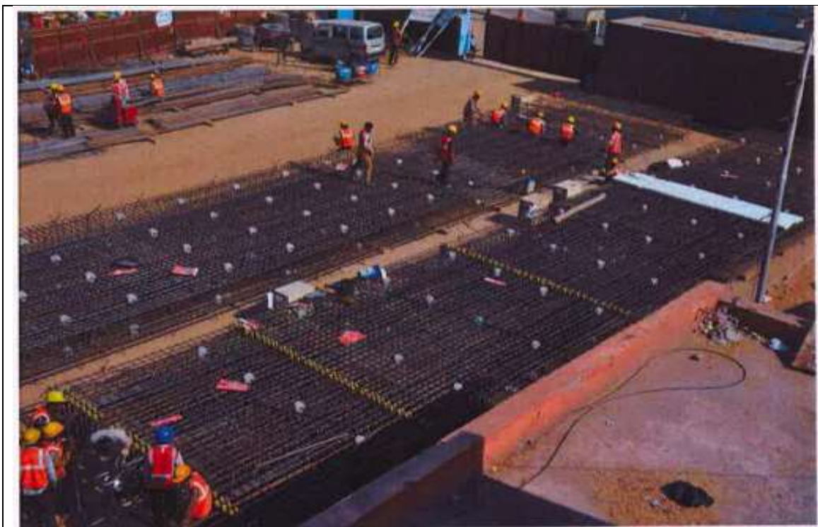
D-Wall Cage Febrication at Chhoti Chaupar
