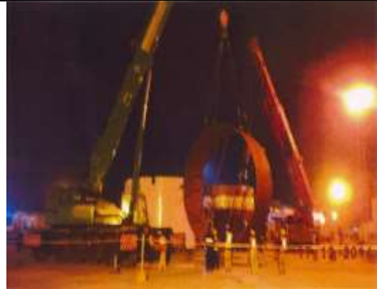
Tilting of TBM-1 Tail Shield
