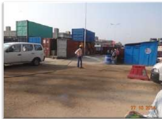
Manual Water Sprinkling at site
