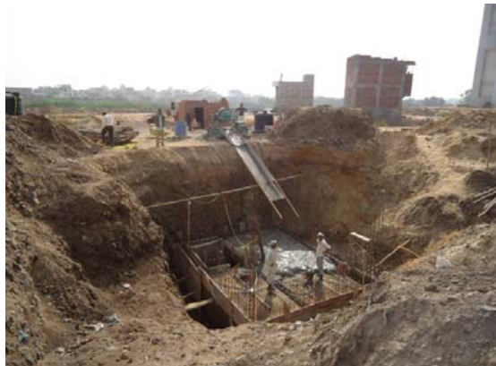
New buildings under construction
