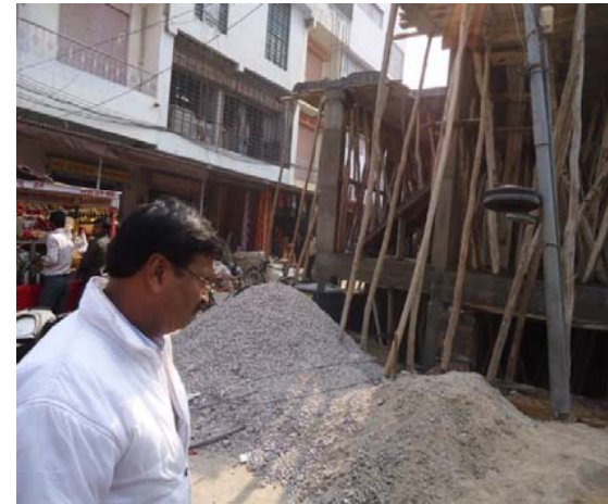
New construction at Sikar House
