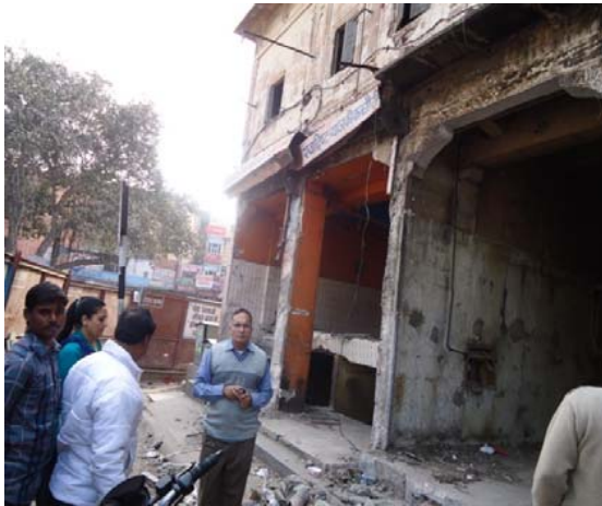
Acquired Shops at Chandpole
