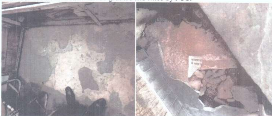
Floor Settlement is observed inside the shop
