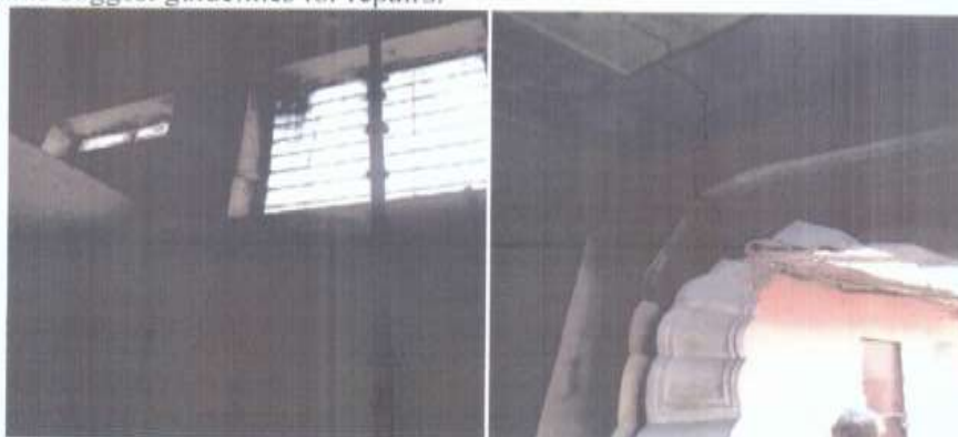
Cracked Masonry Pillar and Arch where propping is required
