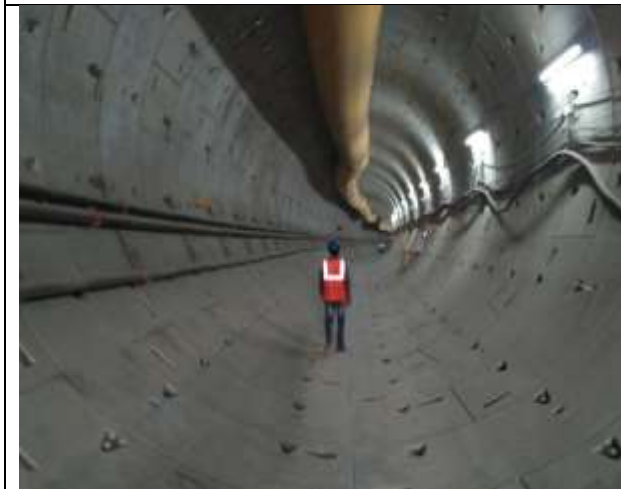
View of TBM-2
