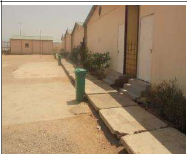
Labour Camp at Casting Yard
