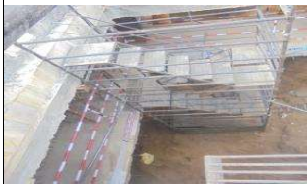
Soil Excavation at Chhoti Chaupar
