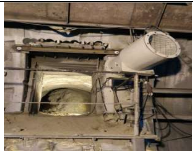
View of cross passage work TBM-1
