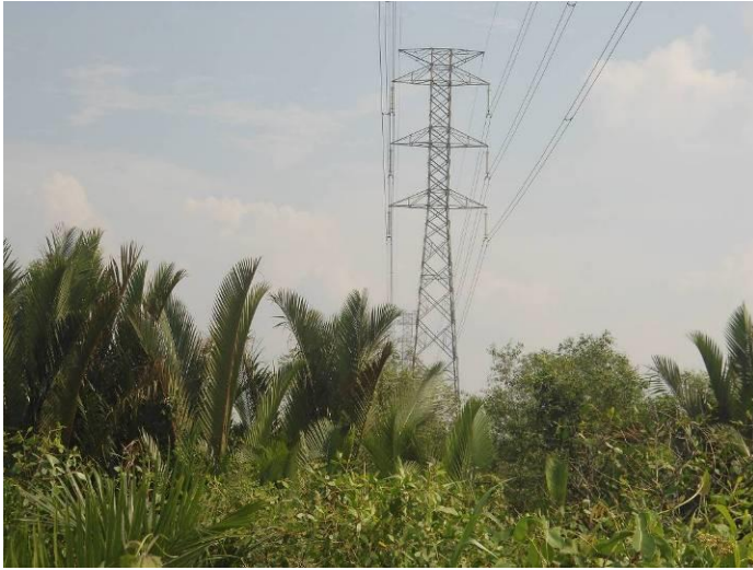
The existing 220kV Cat Lai – Thu Duc T/L
