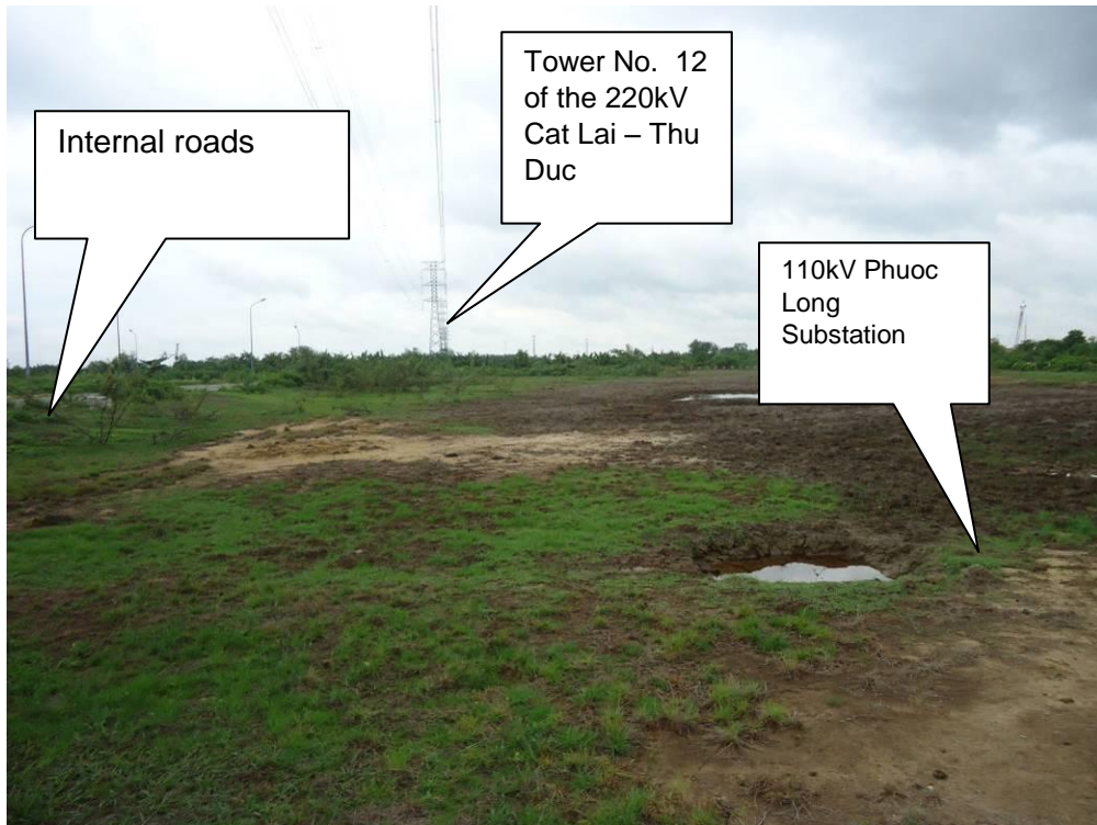
The area projected to construct 110kV Phuoc Long Substation
