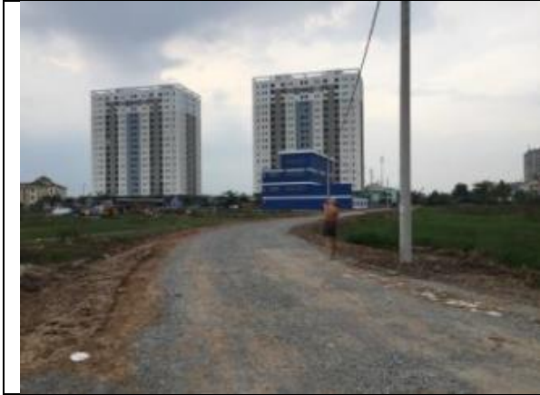
Photo 1: The access road to the new substation has been repaired, upgraded and cleaned
