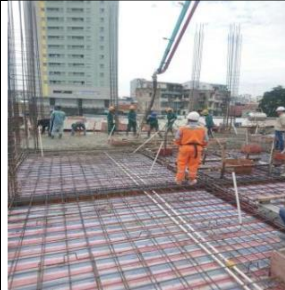
Photo 13: The workers were using proper protective equipment and were provided with satisfactory facilities
