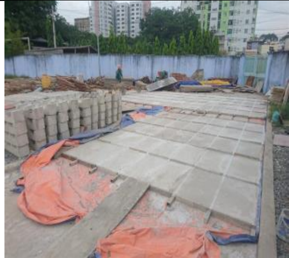
Photo 14: The construction materials are stored or made at separated place in the substation area
