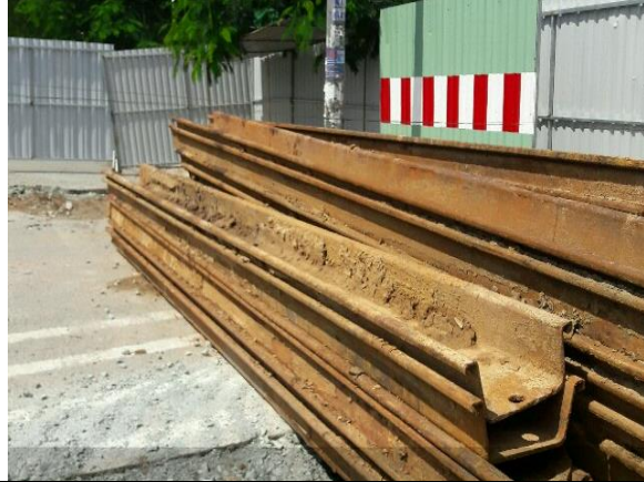
Photo 33: Construction materials were gathered tidy at the site
