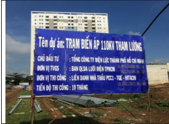
Photo 15: Subproject information board has additional phone numbers of contractors and construction supervision unit
