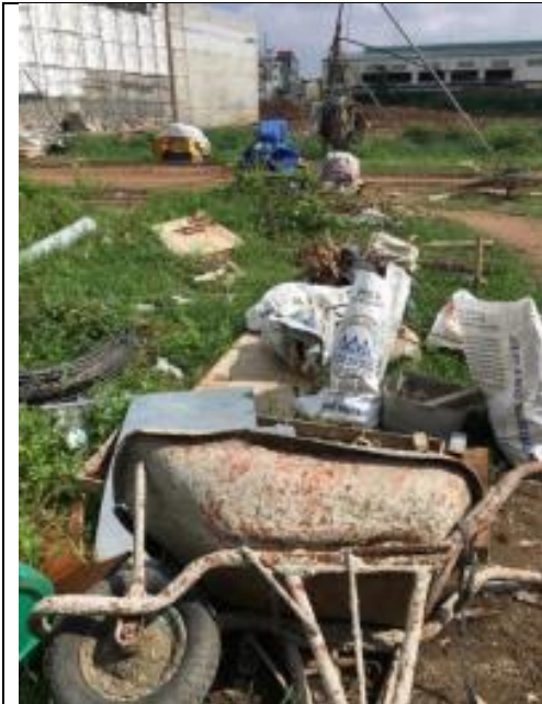
Photo 17: Construction solid waste is not gathered properly
