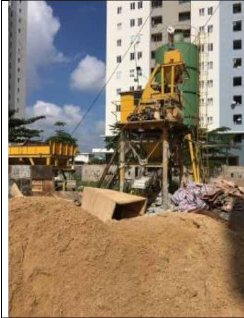
Photo 19: Uncovered excavated soil pile
