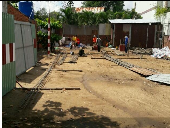
Photo 34: Workers prepared the materials in the fenced construction area
