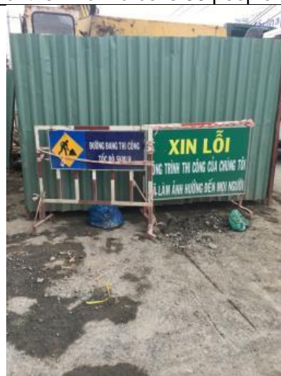
Photo 26: the iron plate fence is surrounding the construction site
