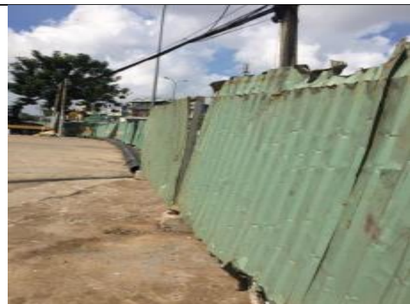
Photo 22: Iron plate fence around the construction area during day time
