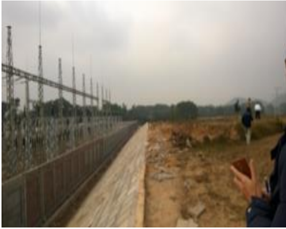
Contiguous area between 220kV substation and location of the first 110kV tower of the sub project
