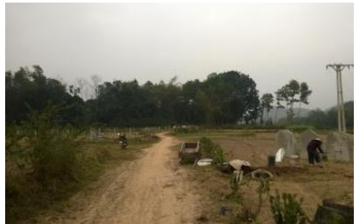
The road to the construction site of feeder column from 220kV substation
