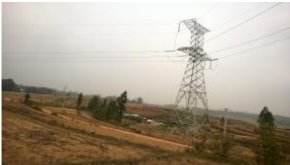
The existing 220kV line, which the newly built 110kV transmission will run parallel with in a distance of about 100m
