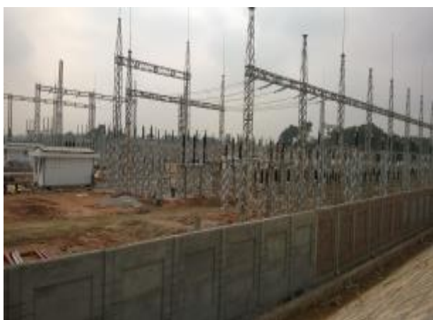
220kV Son Tay substation under construction
