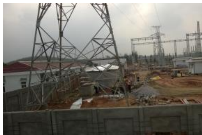
220kV Son Tay substation under construction
