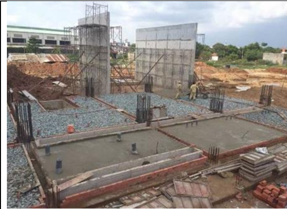
Construction of concrete work on the ground floor bedding)
