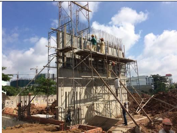
Fire walls (Installation of reinforced wall fire formwork
