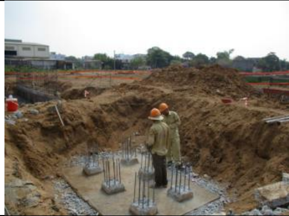
Figure 3: All workers are using personal protective facilities (photo taken 15 April 2016)
