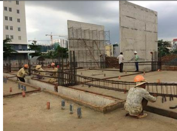
Installation of reinforced beams bracing the ground floor
