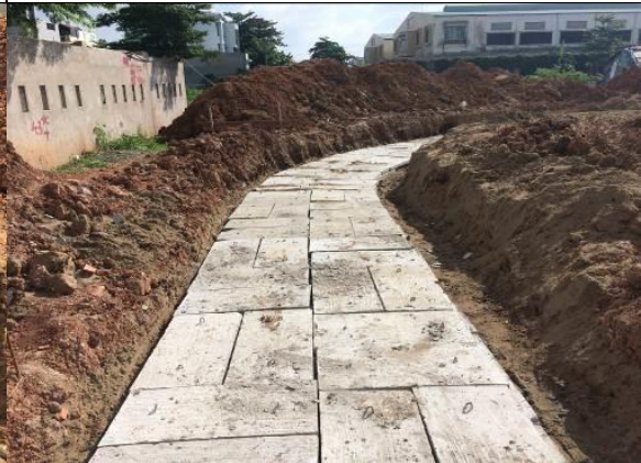
Installation of concrete cable raceways
