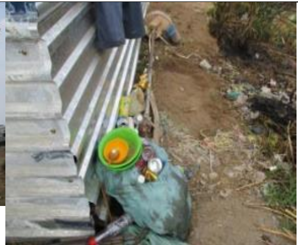
Figure 5: Domestic solid waste at construction site
