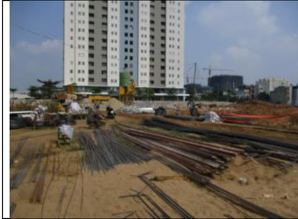
Figure 2: Building materials are gathered in the construction site (photo taken 15 April 2016)
