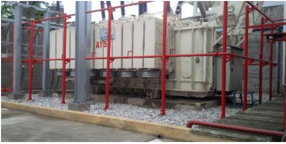
Location at the start of line at Thanh Cong substation
