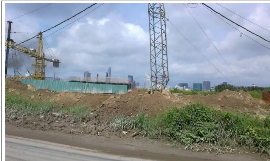
Construction of a bridge on R2 road, ending location of underground cable section to Tran Nao street
