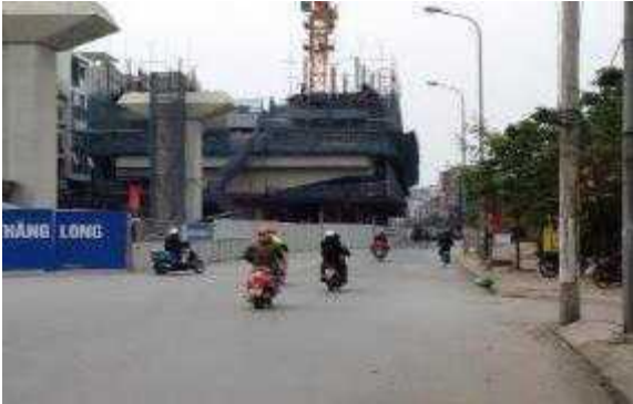
Photo1: The underground cable line runs along Hoang Cau road – Trung Liet ward – Dong Da district
