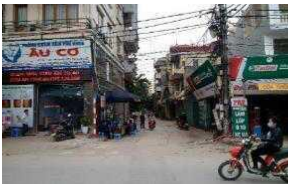
Photo5: Underground cable line runs from beginning of Alley 282 – Khuong Dinh road to the end point of Thuong Dinh substation – Ha Dinh ward– Qthanh Xuan district
