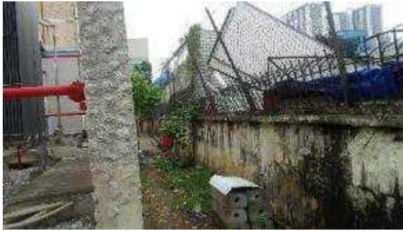
Photo9: Connecting area of Thanh Cong 220kV substation
